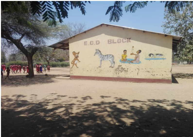
Figure 4.3: School buildings revealing ECD development on the wall
