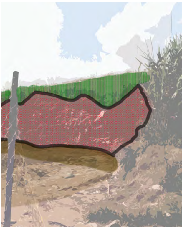
Fig 6.7 Erosion of clay layer to waste layer (Author, 2020)
