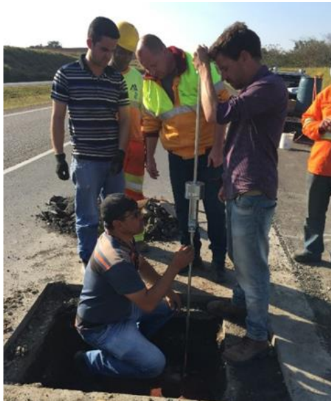
Figure 3-23: Dynamic Cone Penetrometer (DCP) test
