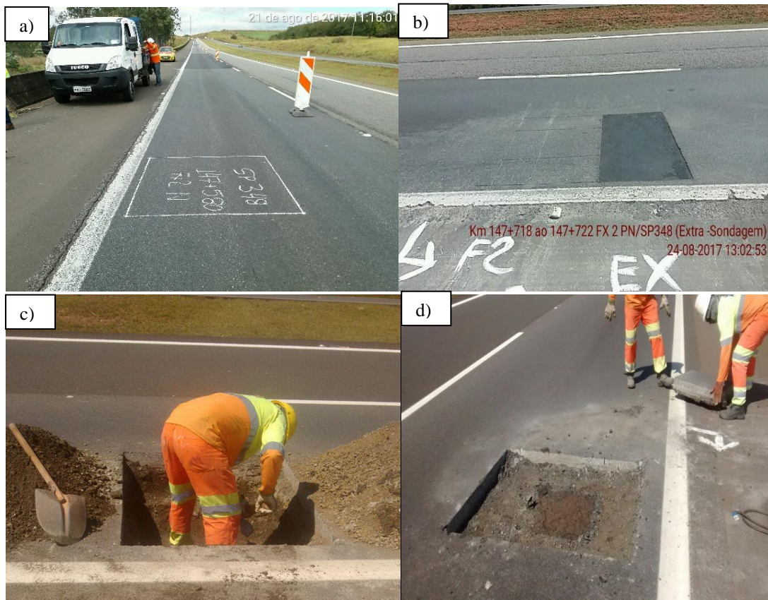
Figure 3-18: a) IP-01 opened in Test Section I b) IP-02 opened in Test Section I c) IP-03 opened in Test Section II c) IP-04 opened in Test Section II
