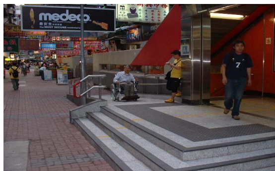
Figure 4. Example of equitable use – ramp and stairs are useful to people with diverse disabilities.
