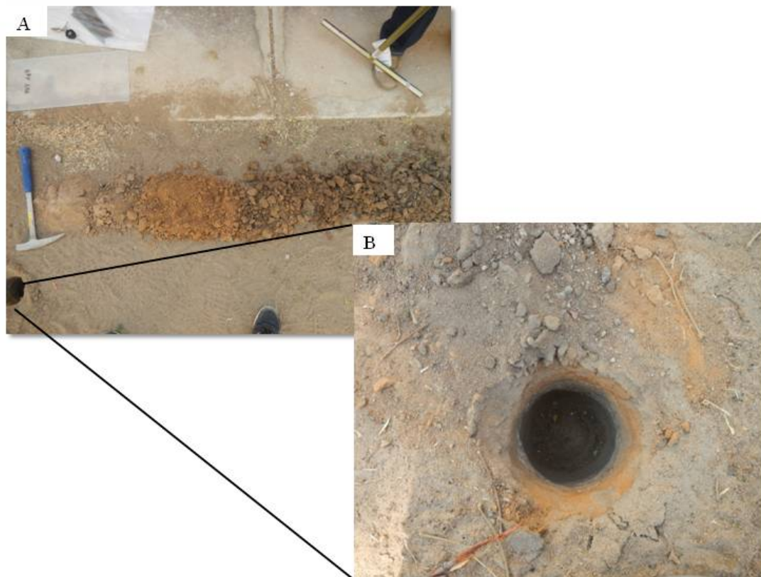
Figure 34: An auger hole in B was developed in the vicinity of a damaged house, showing the red imported sand. This auger hole was profiled, yielding the different soil layers shown in A, with a very distinct red layer of this sand.
