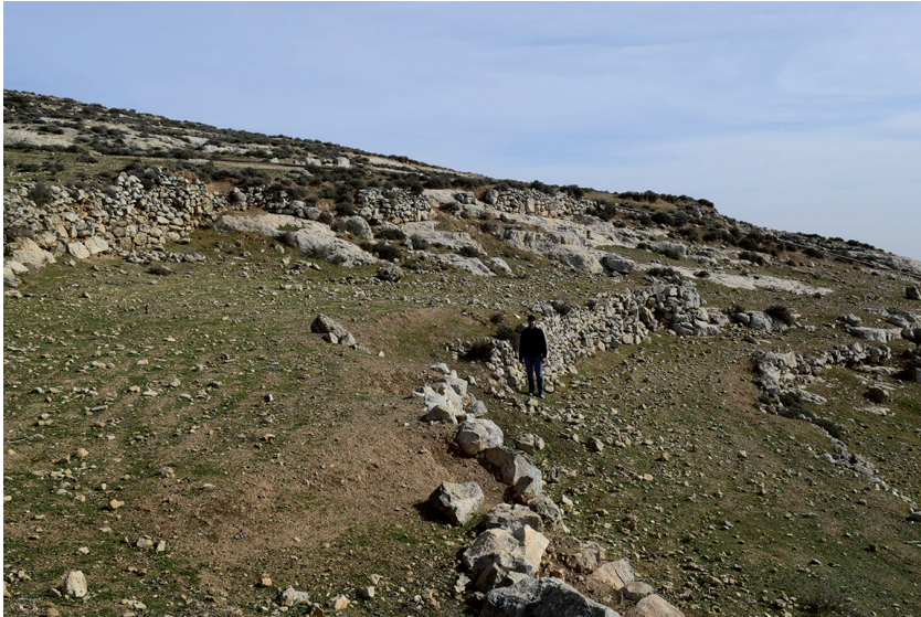
Fig. 16. Retaining Walls, Zone 1 Photo by Robert Miller.
