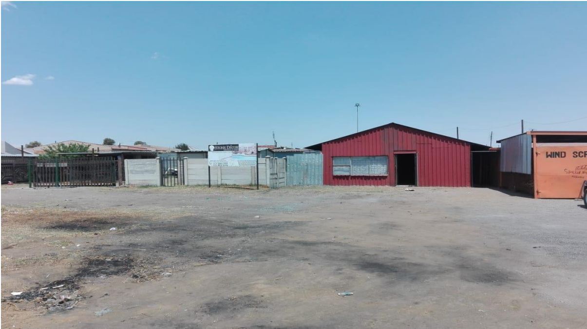
Figure 2. Businesses and a church in eMbalenhle’s main street. Photo credit: RYSE project team.
