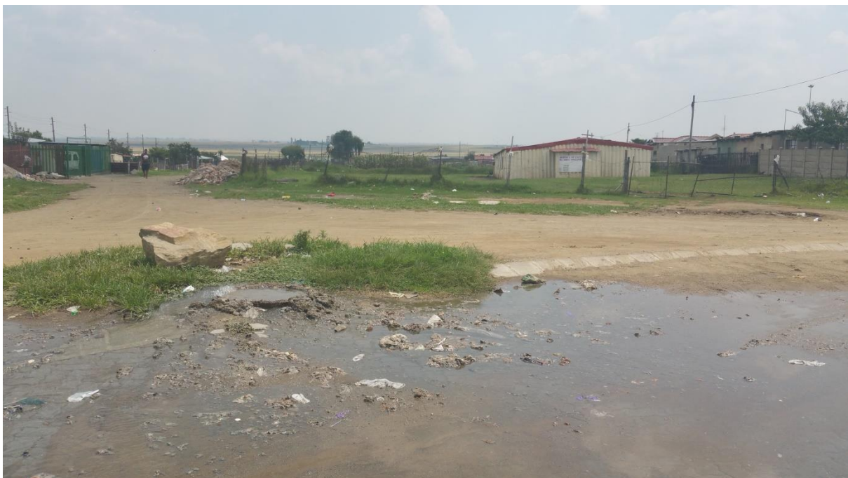
Figure 5. Sewage in eMbalenhle. Photo credit: RYSE project team.
