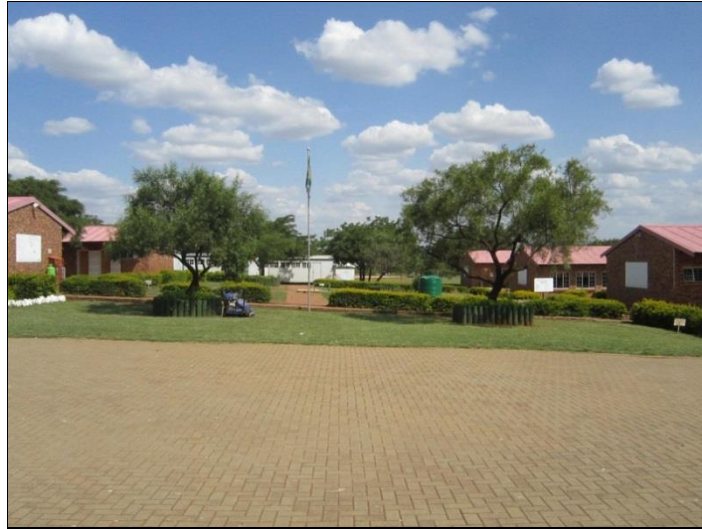
Photograph 3.5 The exterior of one of the schools I visited
