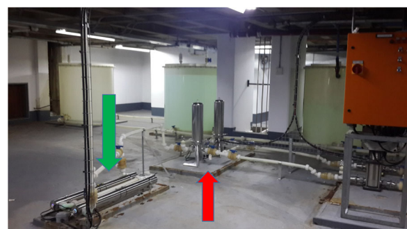
Fig. 3 Series of filters (red arrow) past the reverse osmosis pump and 2 UV lights (green arrow) which is the final sterilisation step prior to water entering the wards
