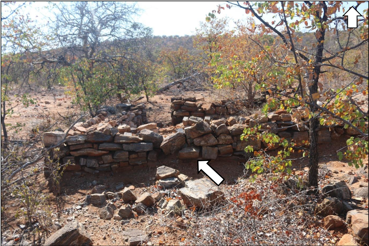
Figure 5.77: Evidence of a break in east wall of the stone enclosure.
