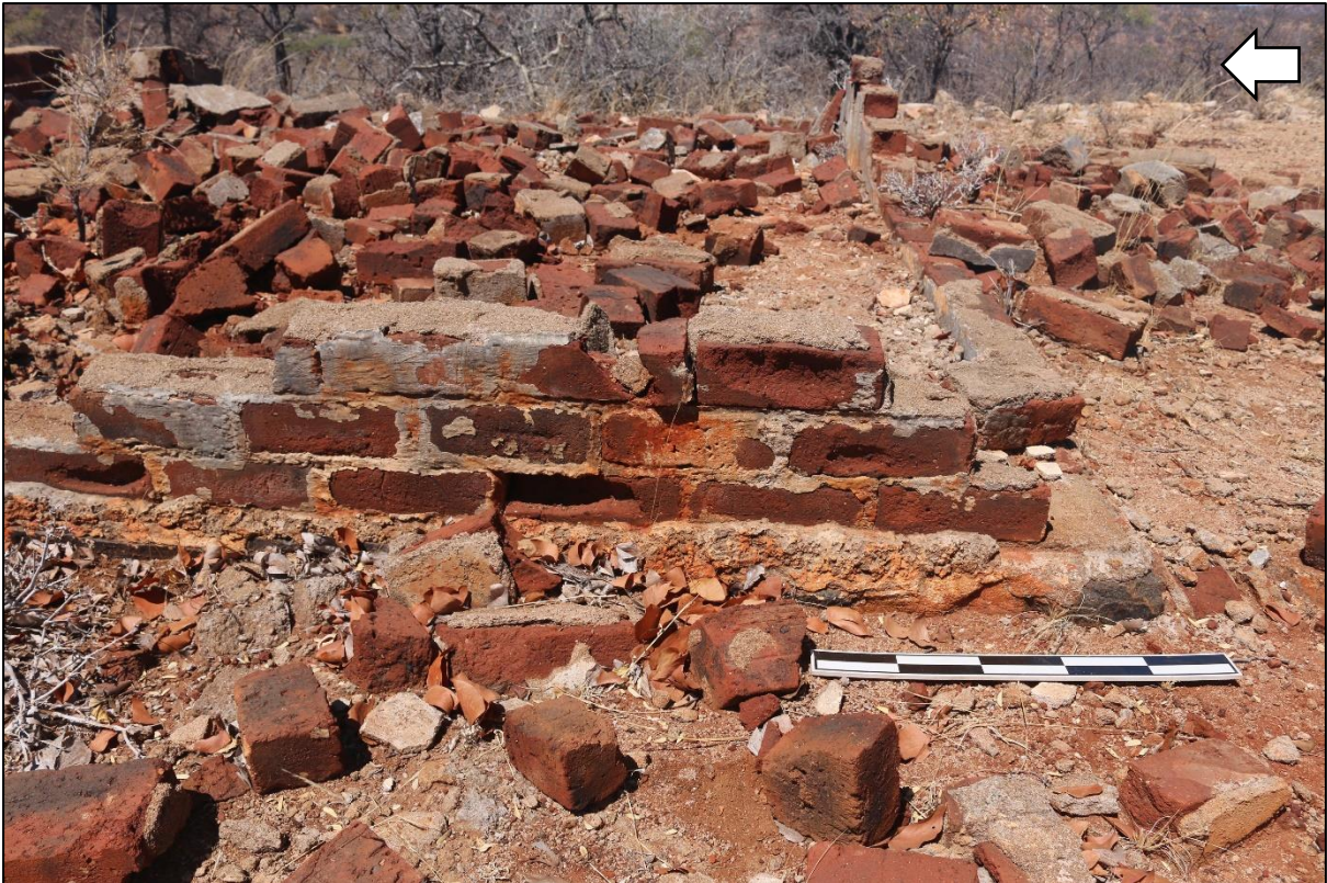
Figure 5.67: Foundation of Building 2 with red brick wall built on top.
