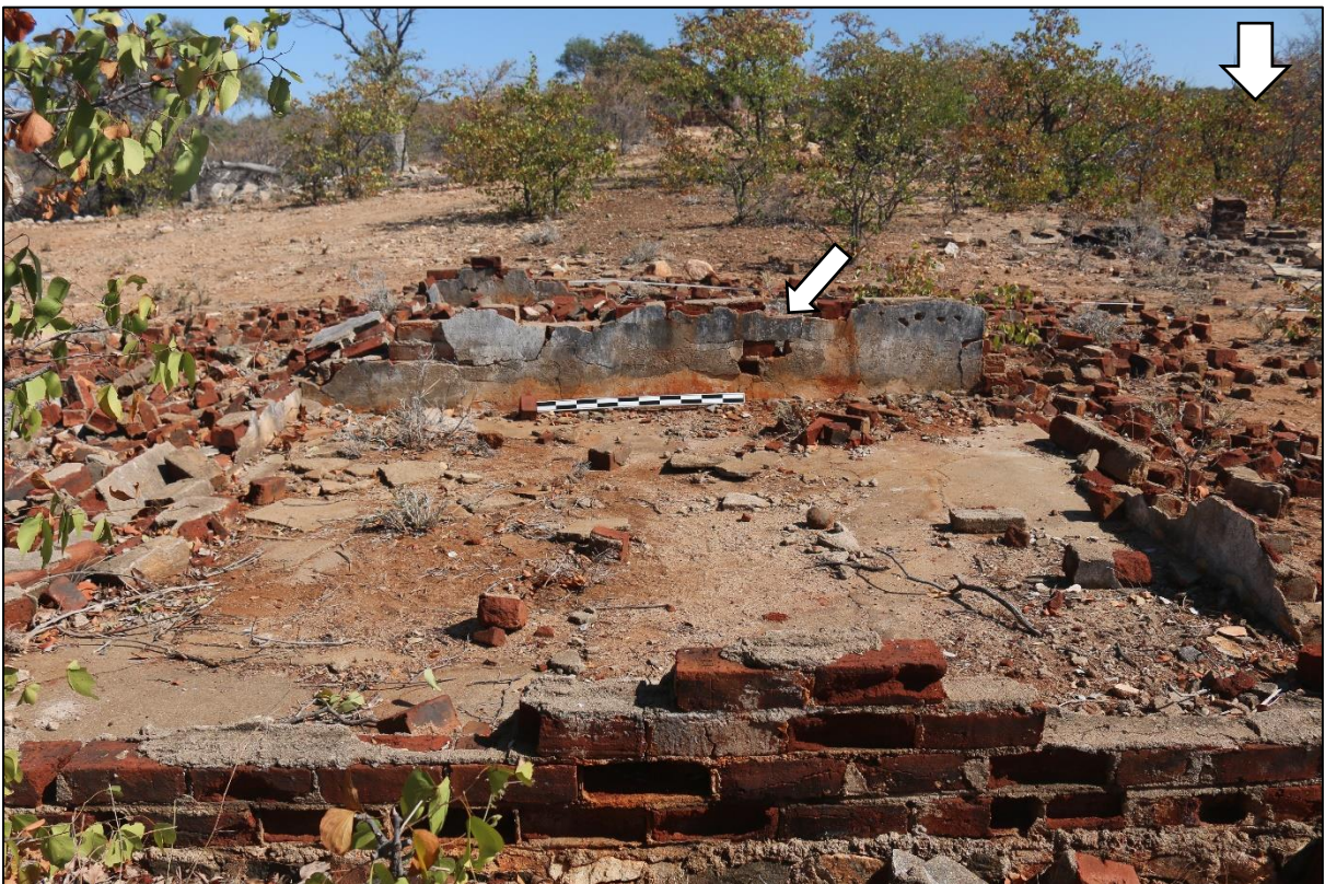
Figure 5.69: Dividing wall of Building 2, which includes plaster on inside of the wall.
