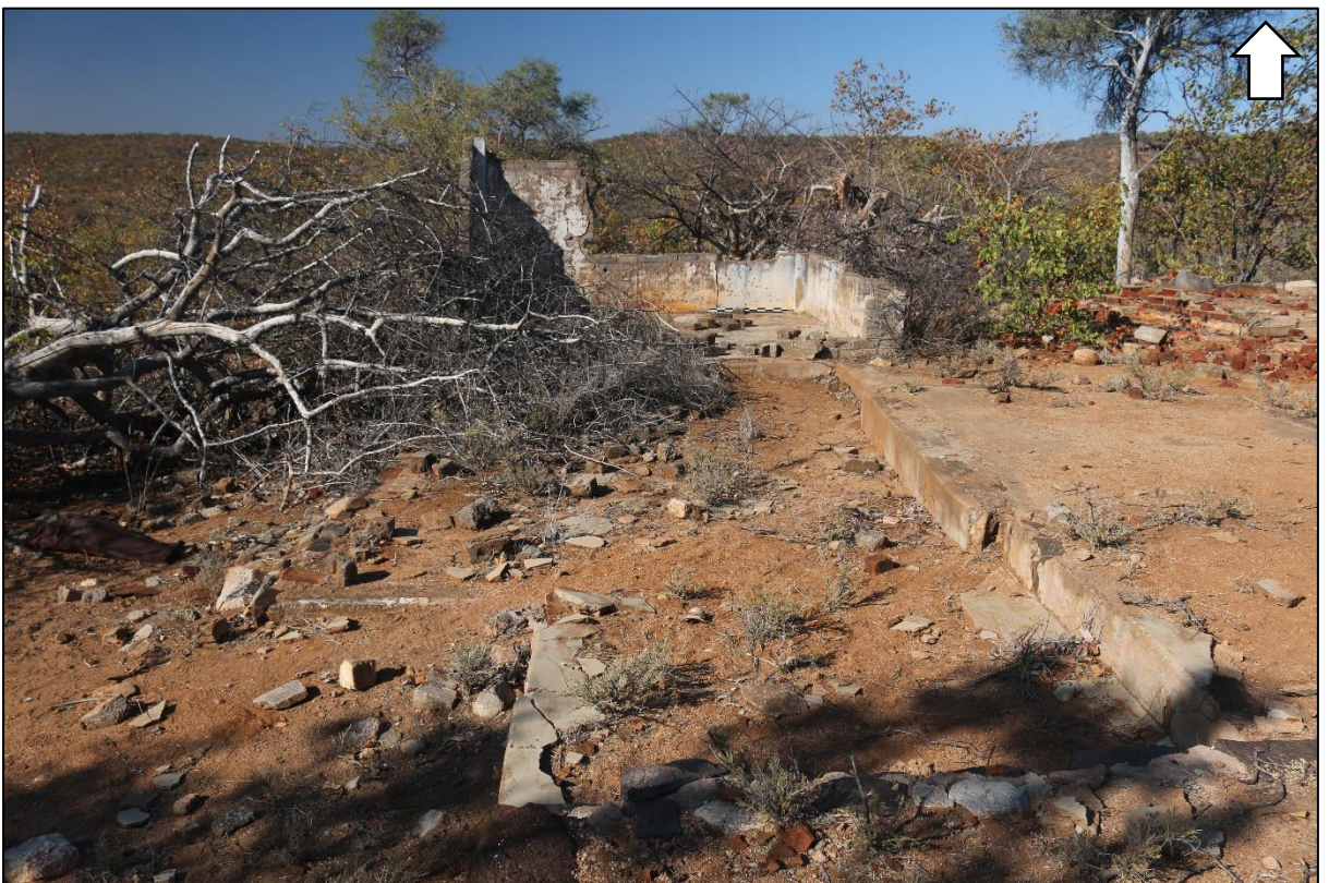
Figure 5.34: Building 1 (grey brick and stone building). Area C and B.
