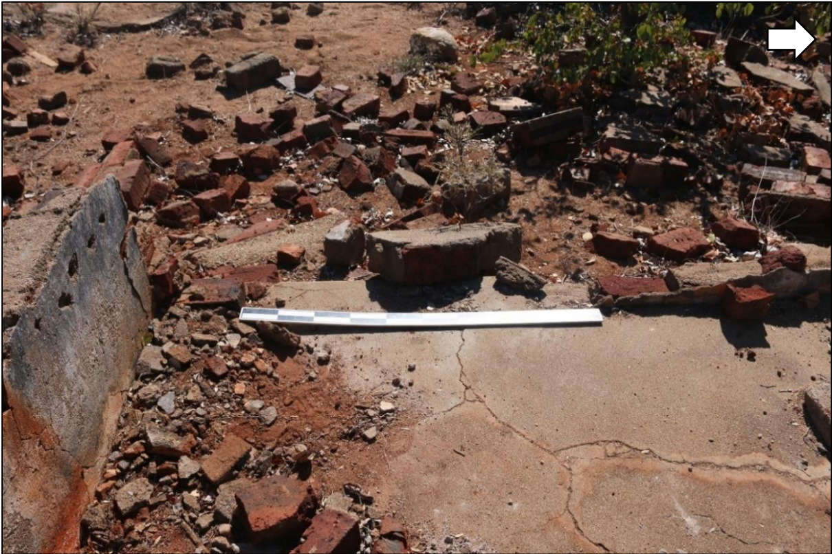
Figure 5.66: Entryway (room 2.2) located at Building 2.
