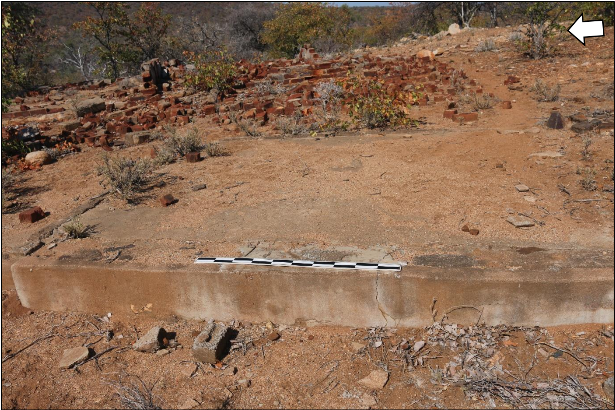
Figure 5.39: Close-up of inside stone foundation covered in concrete of Building 1. Area C.
