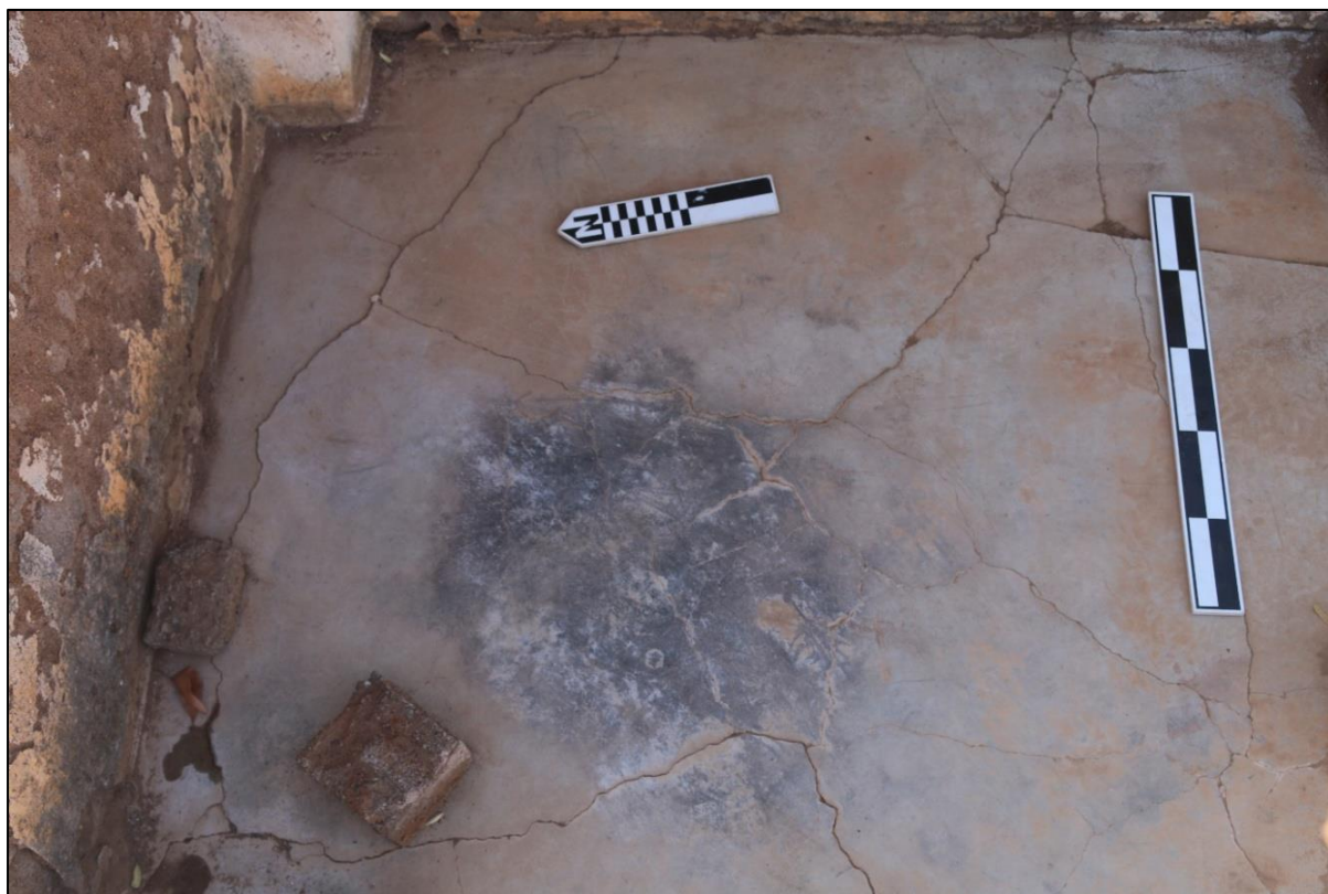
Figure 5.52: Burnt patch on the floor on the inside of Building 1 in room 1.1. (Area B).
