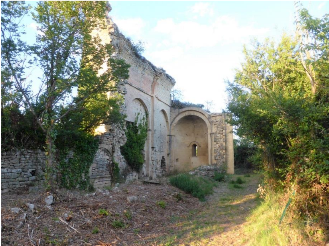
4Ruins of St Christophe, near Avignon, destroyed in the 14th century during the fight of the church against heretic communities Photo: H Müller
