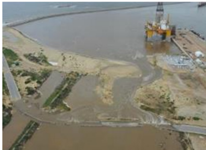
Figure 7: View of the Coega River flood towards the sea (TNPA, 2011b)
