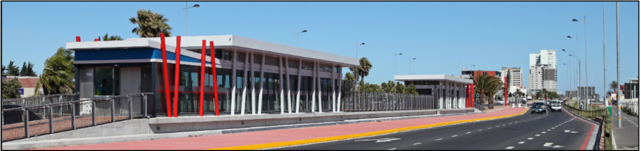
Figure 1: MyCITI station in Cape Town (HHO, 2018)
