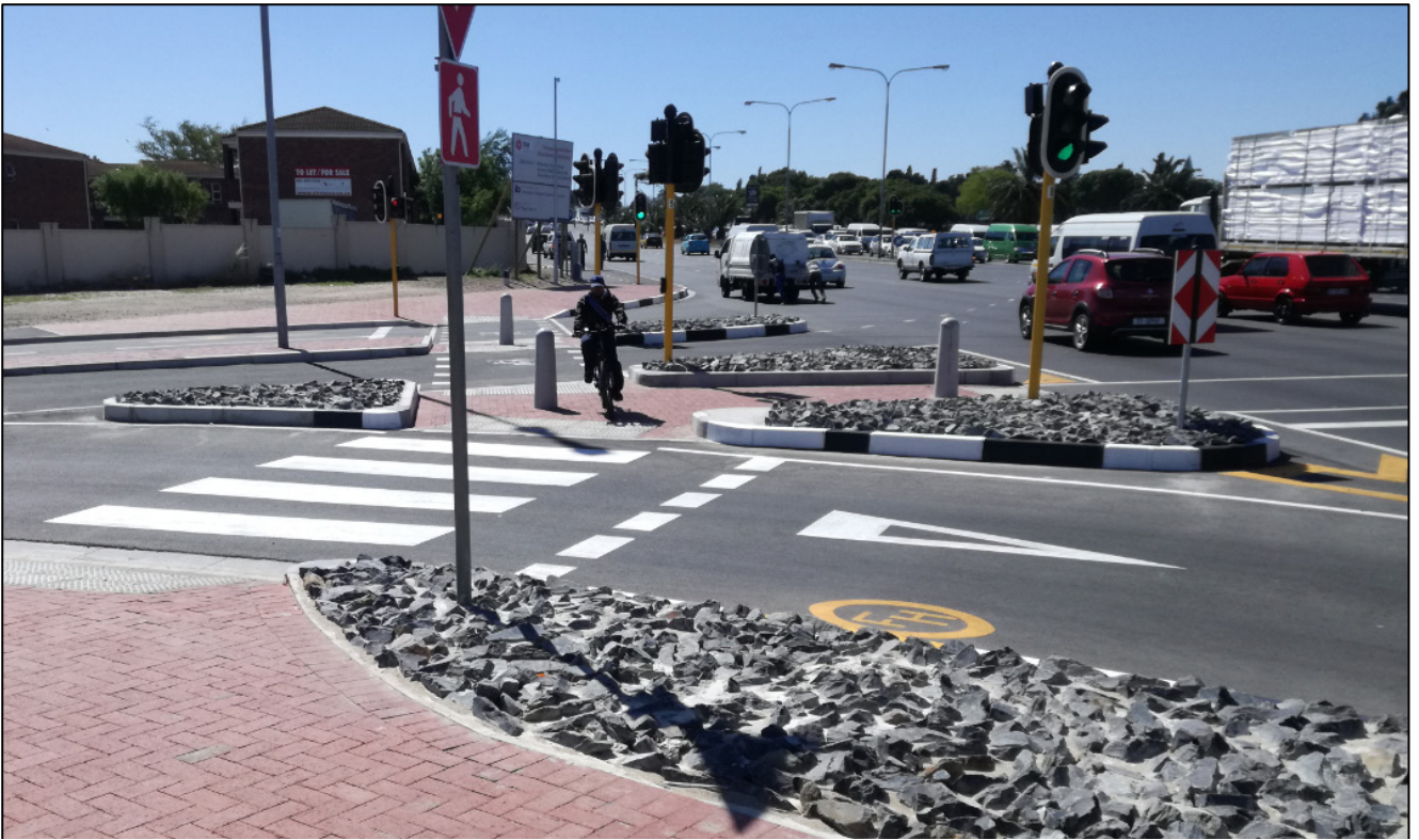
Figure 9: Pedestrian cycling facilities – Note detail of level crossing, channelisation and stone pitching
