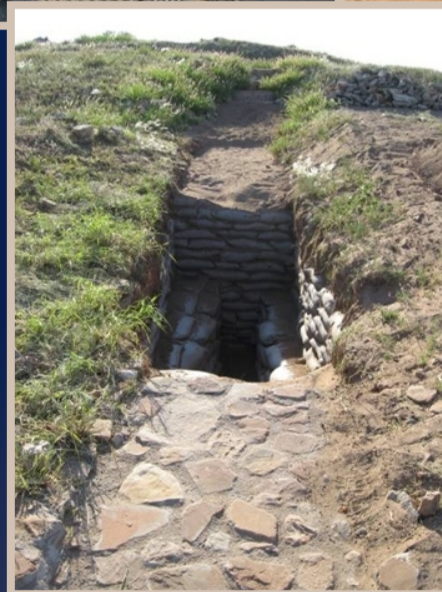
Figure 4: Re-burial site on Mapungubwe hill (Jones-Schofield 1934 Trench 5) illustrating the sandbag stabilization underneath the walkway
