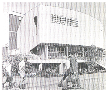
The Aula, main entrance and south-east elevation.
