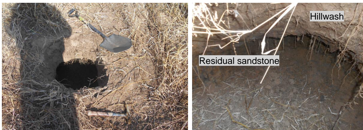
Figure 3-12: The partially collapsed sinkhole at TP02.
