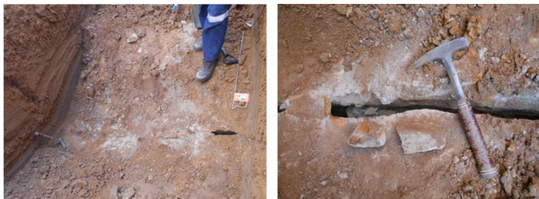
Figure 3-22: Crack in the rock at TP06 covered with sandstone and open below.
