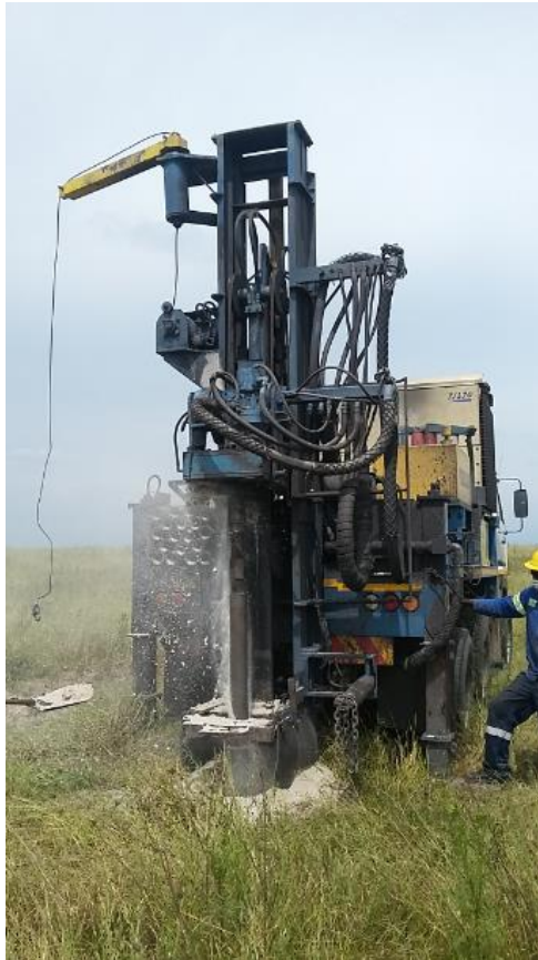
Figure 3-9: Percussion borehole rig drilling BH01.
