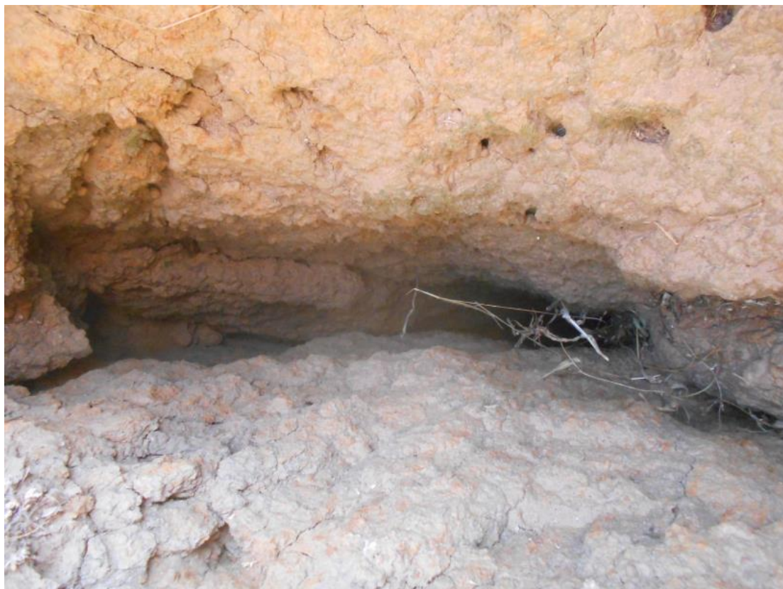
Figure 3-21: Looking down into the empty V-shape of the sinkhole at TP06.
