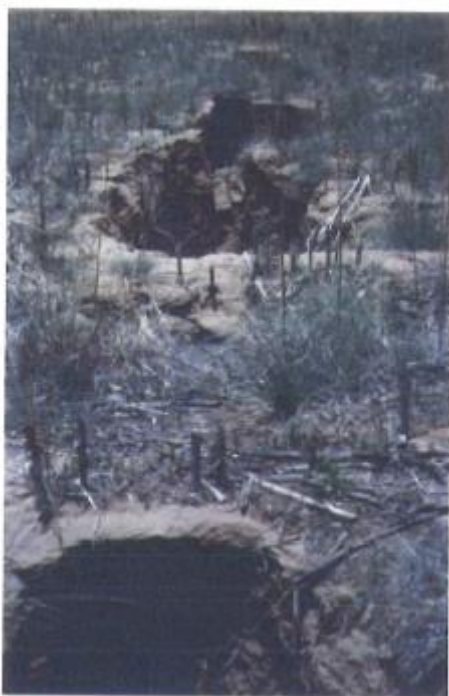
Figure 2-3: Strip like sinkholes with the soil arch above the subterranean tunnel (Van der Merwe, 1990).
