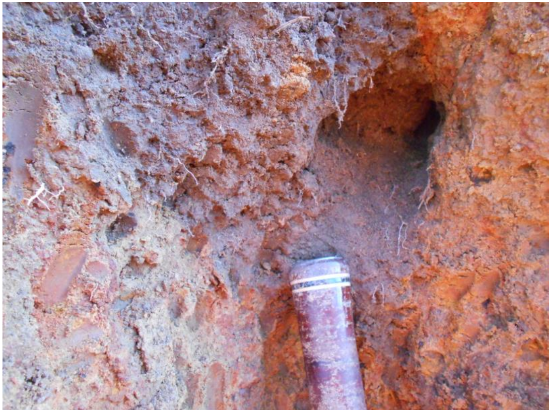
Figure 5-14: Termite activity within hillwash infilled crack in residual sandstone at TP10.
