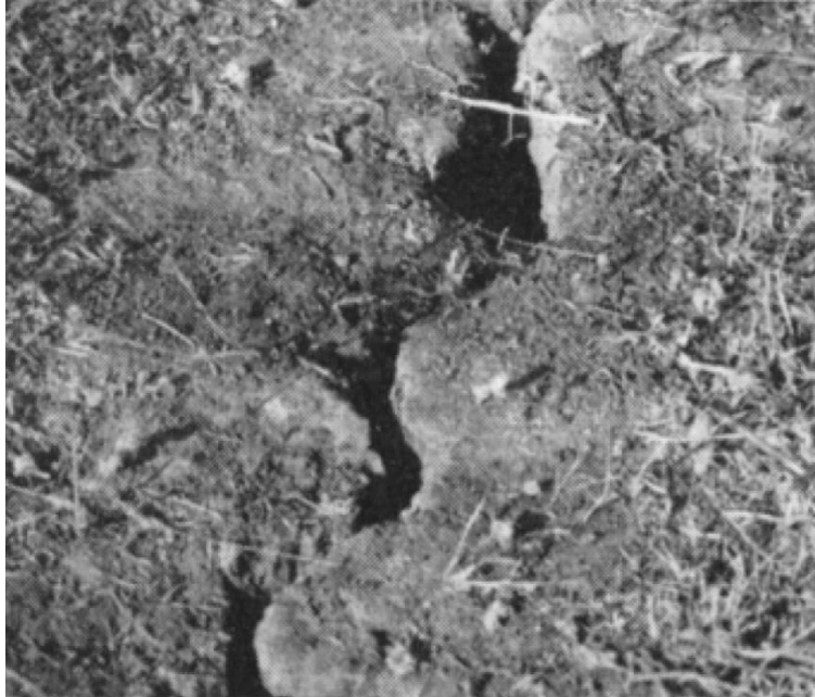
Figure 2-17: Shrinkage crack in cultivated field (Marr, 1955).
