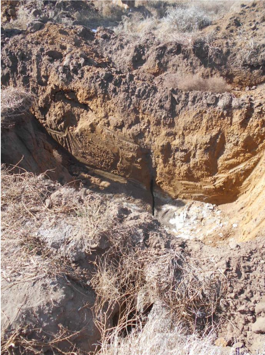
Looking east across TP04 and TP05, showing the excavated crack in the rock, infilled V-shape and small sinkhole on surface in the foreground.
