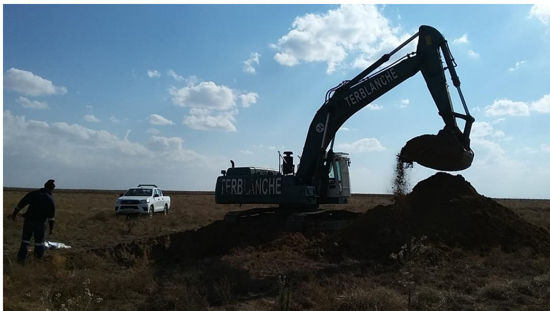
Figure 3-7: 20 ton excavator excavating at TP06.
