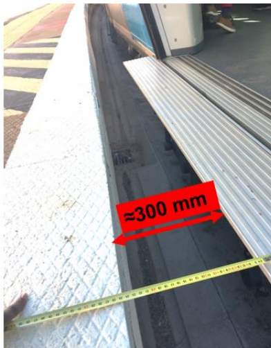
Figure 3-22: Walker street station
