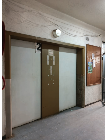
Sealed elevator shafts
