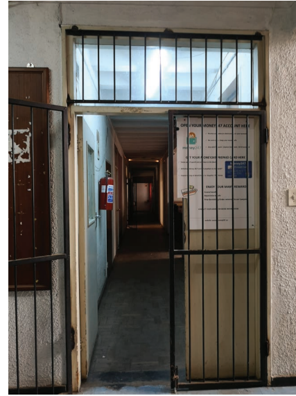
View down southern passage
