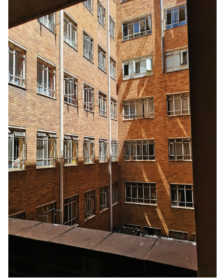
View into light well
