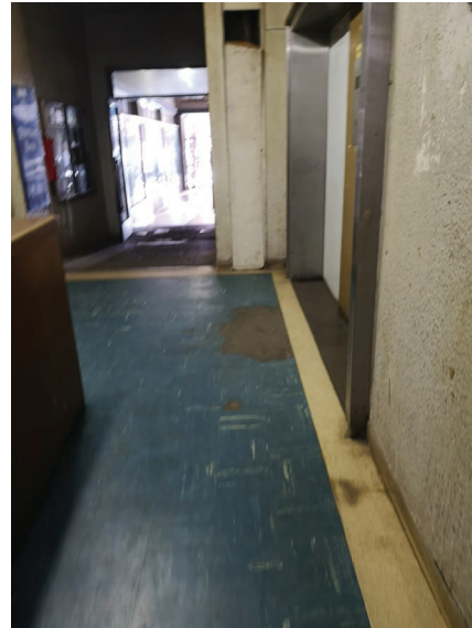
Ground floor lift lobby area
