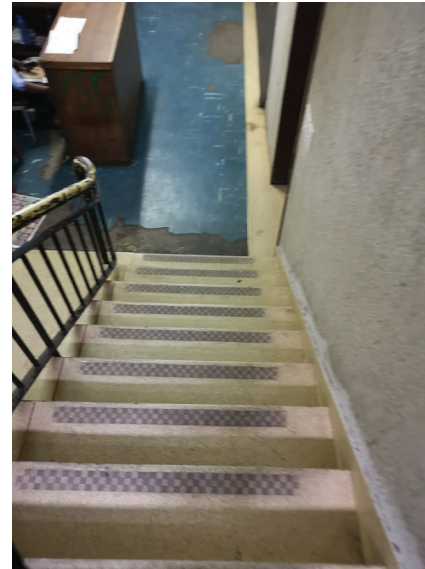
View down stairwell to ground floor
