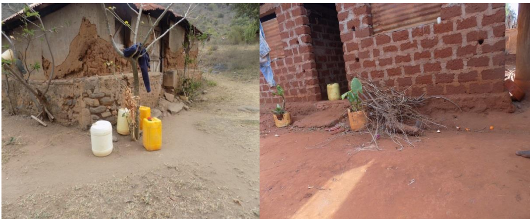
Figure 7.7: Photographs of a dilapidated house and an ordinary house
