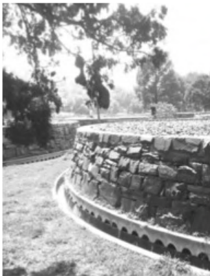
Original 1913 biofilters (Renton, 2018)
