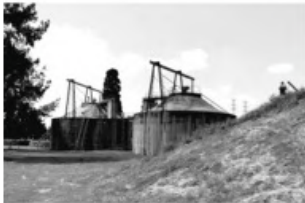
Settling tanks covered in algae (Renton, 2018)
