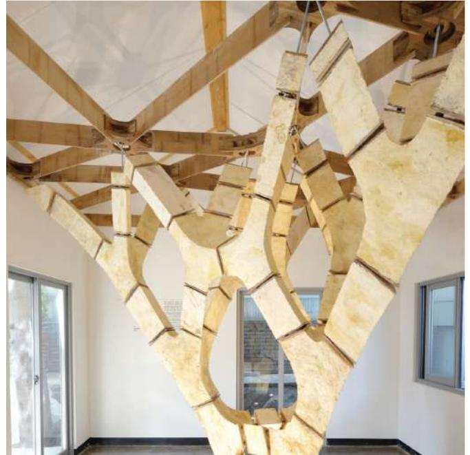
FIG 6.27 & 6.28 : Completed mycelium self-supporting structure (Aouf, 2018).
