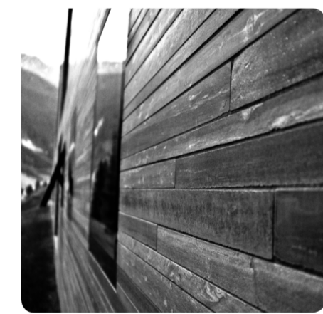
Figure 6.36 - Strictly ordered stonework
