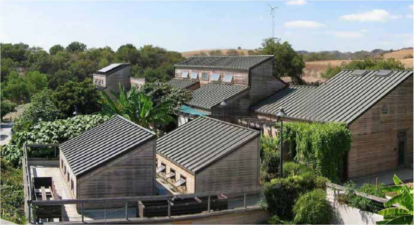
Fig. 18 Top: Perspective view of the Lyle Centre for Regenerative Studies (Cal Poly Pomona, 2019)
