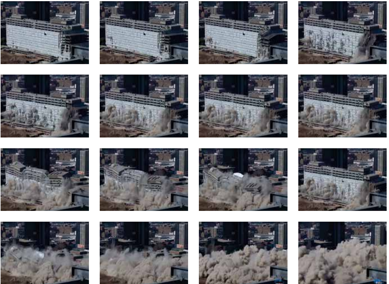
Fig. 1 Top: Demolition sequence of the Munitoria building (ENCA, 2013)
