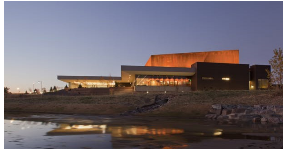
Fig. 5.10 Exterior view of PACE (Semple Brown, 2013).
