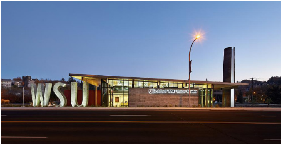
Fig. 7.4 (top) WSU Centre view from the east piazza (Olson Kundig,2013)
