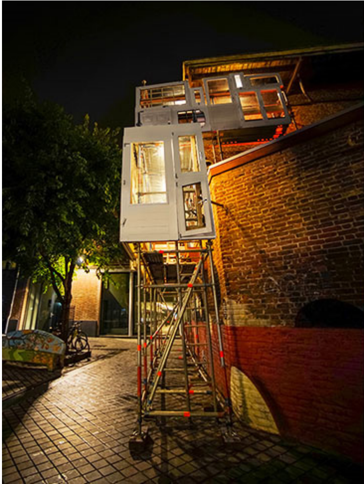
Fig. 5.16 Close up view of Bow House (Malka, 2014).
