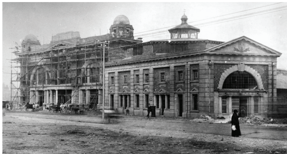
Figure_76 Historic photograph of the Market Theatre being built (The Market Theatre Foundation, 2018)
