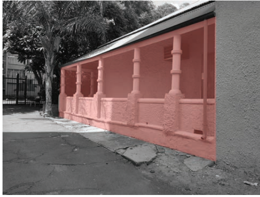
Figure_39 Northern balcony of Heritage house at Breytenbach Theatre
