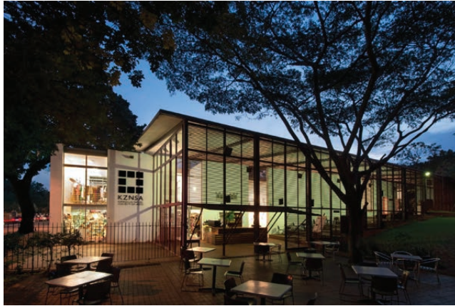
Figure_79 KZNSA Gallery facade (Walters and Cohen Architects, 2000)
