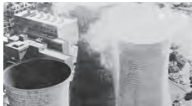
Figure 41: Completion of Cooling Tower (Unknown, 1998)
