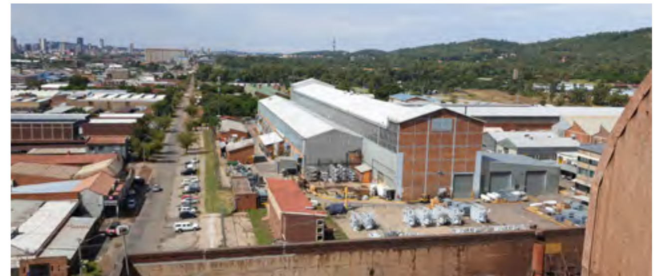
Figure 27: SGB_Smit Power Malta
