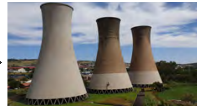
Figure 45: Current State of Cooling Tower
