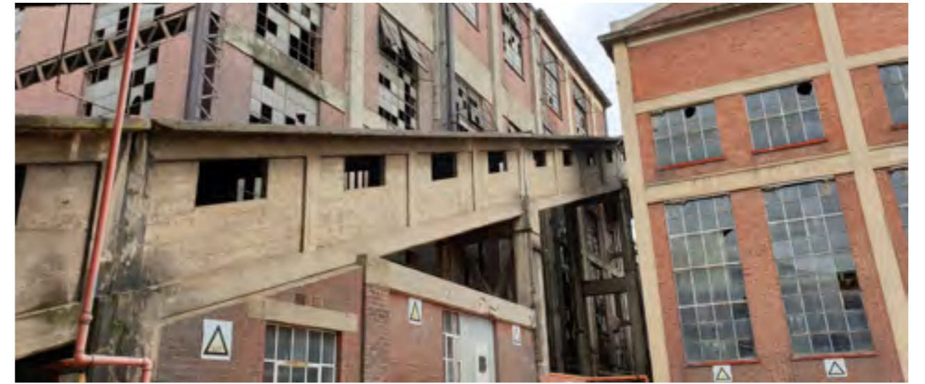
Figure 26: 1942 Power Station (A)
