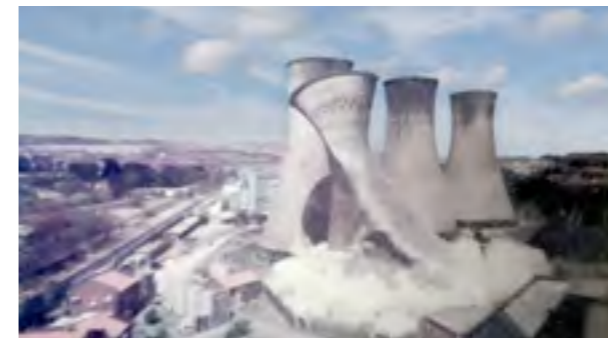
Figure 44: Demolition of Cooling Tower
