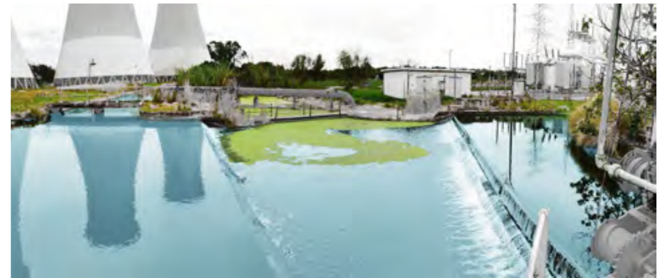
Figure 33: Water Infrastructure - View from existing CW. Pump Room
