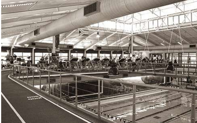
Fig.108: The multipurpose gym with swimming pool below (Sports Science Institute of South Africa: 2019)
