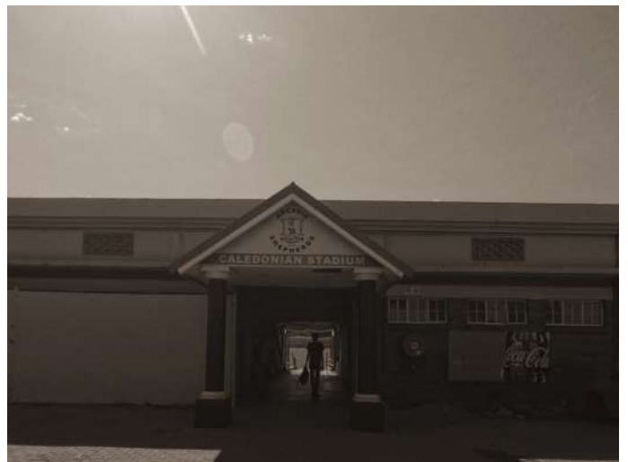
Fig.68: Photo of the tunnel running onto the field (Author: 2019)
