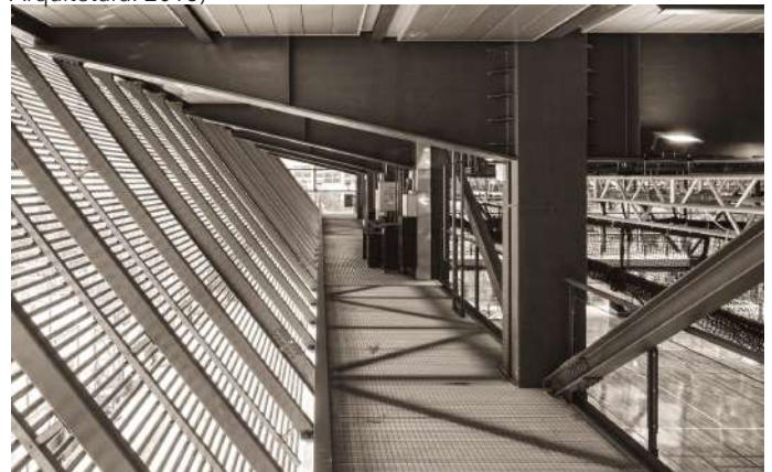
Fig.113: Natural ventilation allowed through shading devices (Urdi Arquitetura: 2016)
