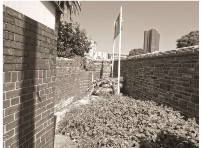
Fig.67: Photo of the old public changing rooms (Author: 2019)
