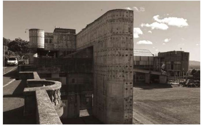
Fig.114: The facade facing the rugby field (Bell: 2012)
