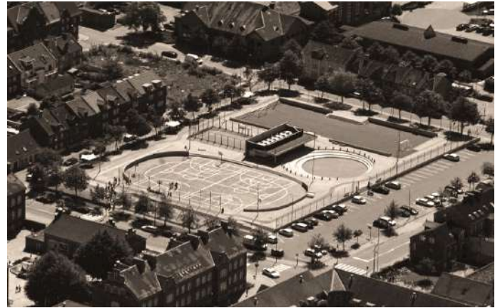
Fig.98: Aerial image of the site intervention (Visitlillebaelt: 2017)
