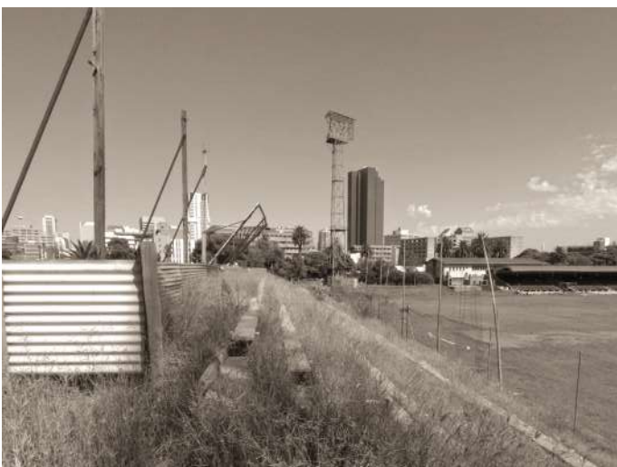
Fig.66: Photo of the southern stands with lack of maintenance (Author: 2019)
