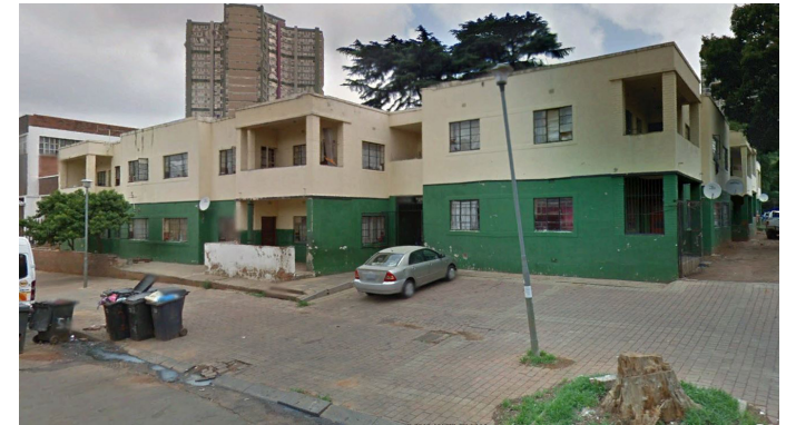
Figure 4-29: Residential building north of railway line
