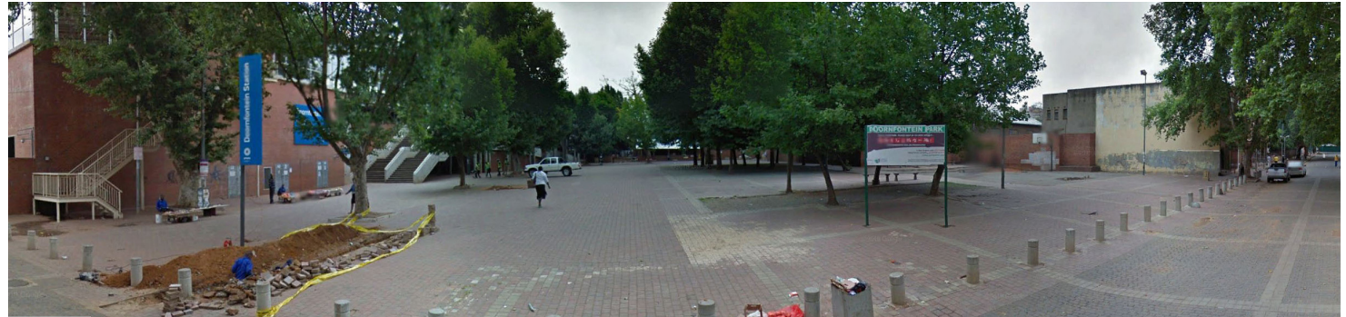
Figure 4-57: Site analyses - Photo analyses, corner of Currey street and Buxton street showing empty plaza, defined by low density buildings with dead edges (Author, 2019)
