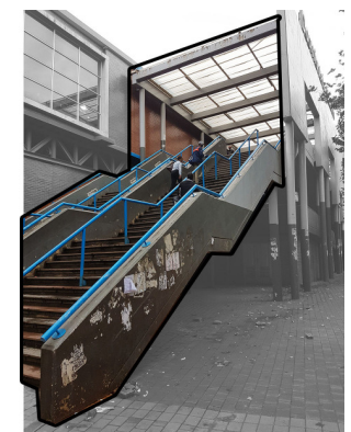
Figure 4-37: Staircase access to station from the station plaza (Author, 2019)
