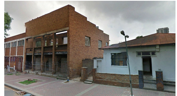
Figure 4-28: Abandoned building north of the railway line
