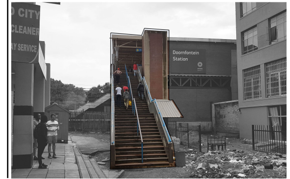
Figure 4-34: Site analyses - Station staircase on Davies street. (Author, 2019)
