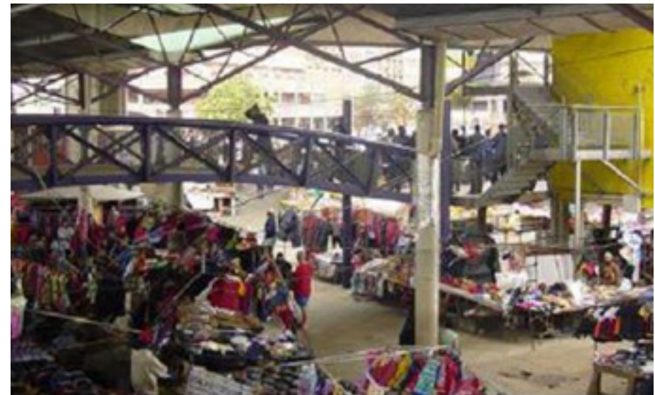
Figure 37 the covered market space (Dobson, 2001)
