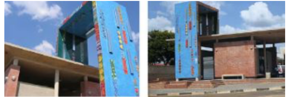
Figure 39 entrance as prominent focal point
