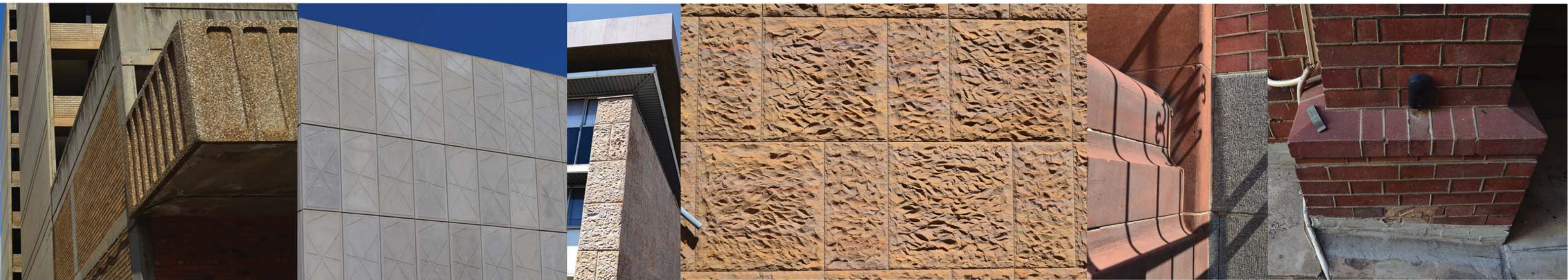
Multiple concrete elements
