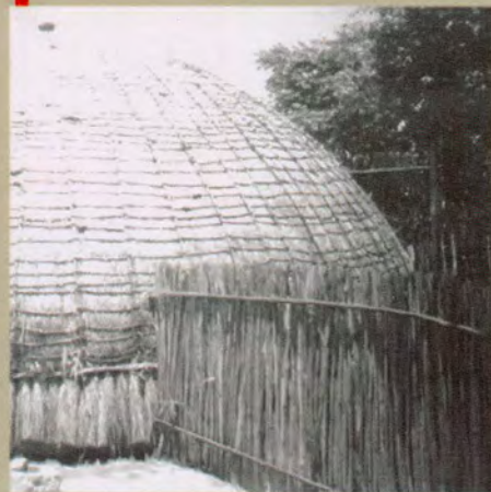
Figure 66 early fencing structure
