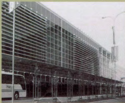
Figure 87 CICC street view
