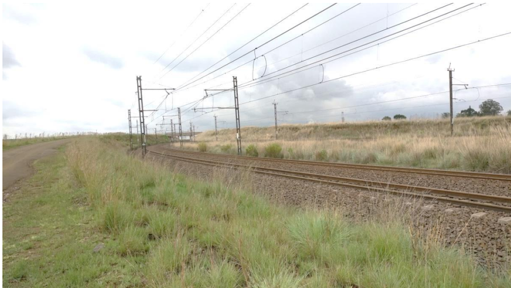
Figure 4-2: Instrumented section of track; view towards South-Western direction
