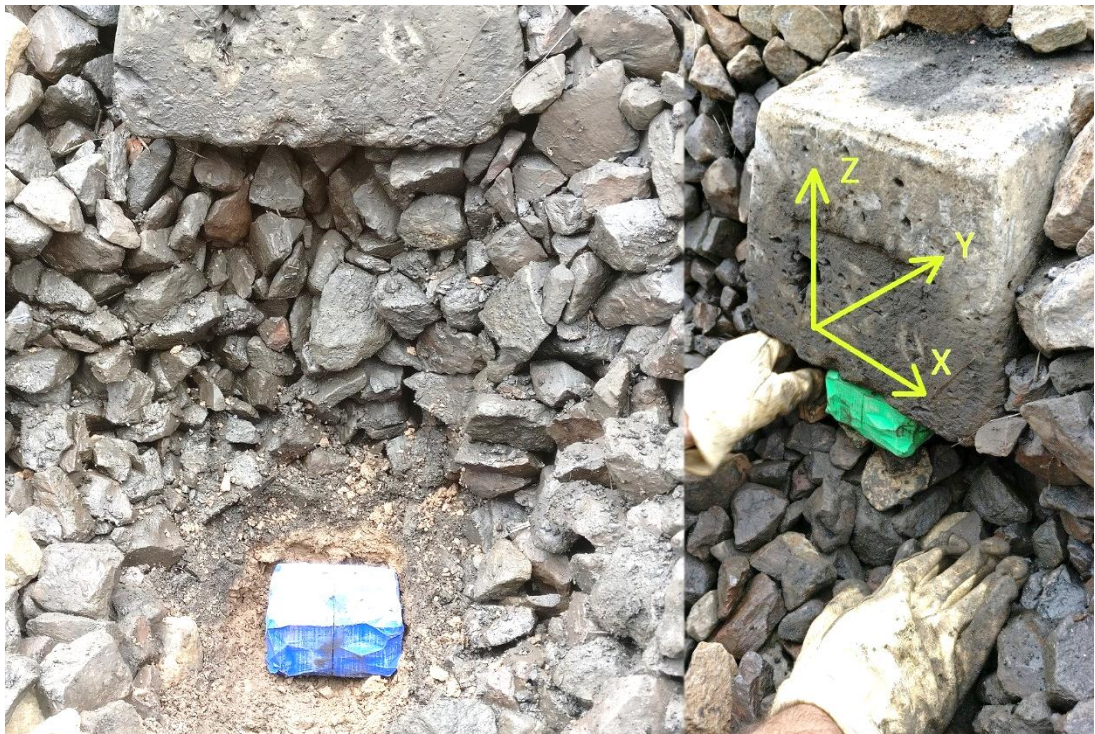
Figure 4-3: Installation of Kli-Pi 1 and 3 just below the ballast and sleeper respectively
