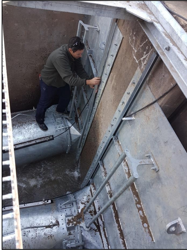
Figure D-9: Covering of the exposed turbine wiring
