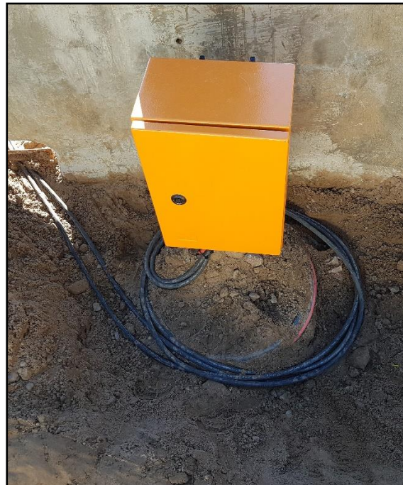
Figure D-10: Electricity box connecting the turbines and the powerhouse, located next to the intake structure.
