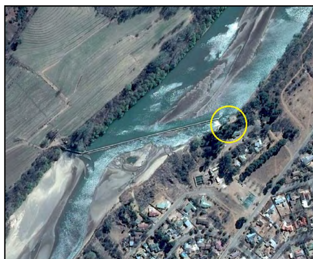
Figure 5-2: The Decommissioned Hydropower Plant Along the Weir at Aliwal North.
