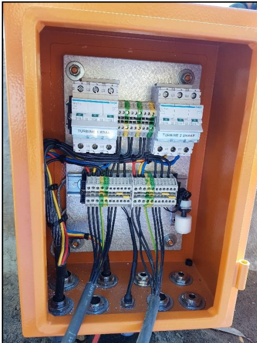
Figure D-10: Electricity box connecting the turbines and the powerhouse, located next to the intake structure.
