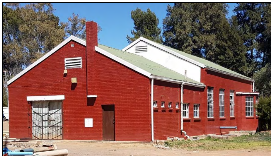
Figure 5-4: Powerhouse at Aliwal North
