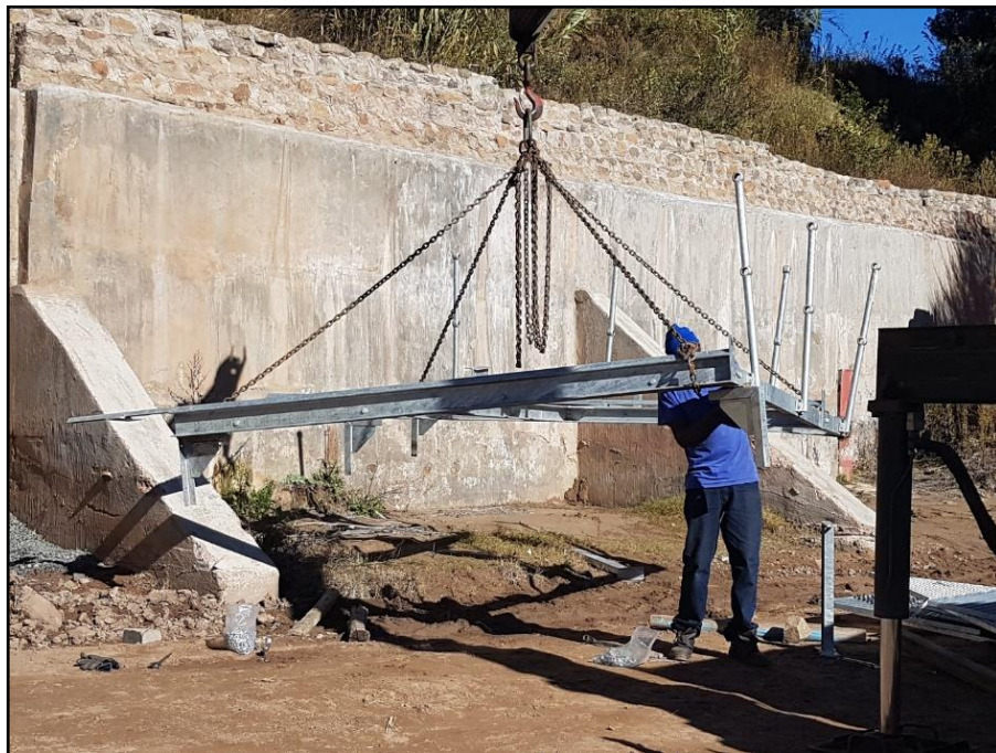
Figure D-2: Assembly of the new walkway
