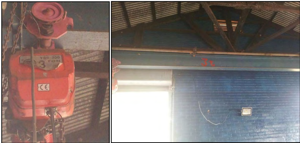
Figure 5-5: The 3-ton Crane and Crawler Beam
