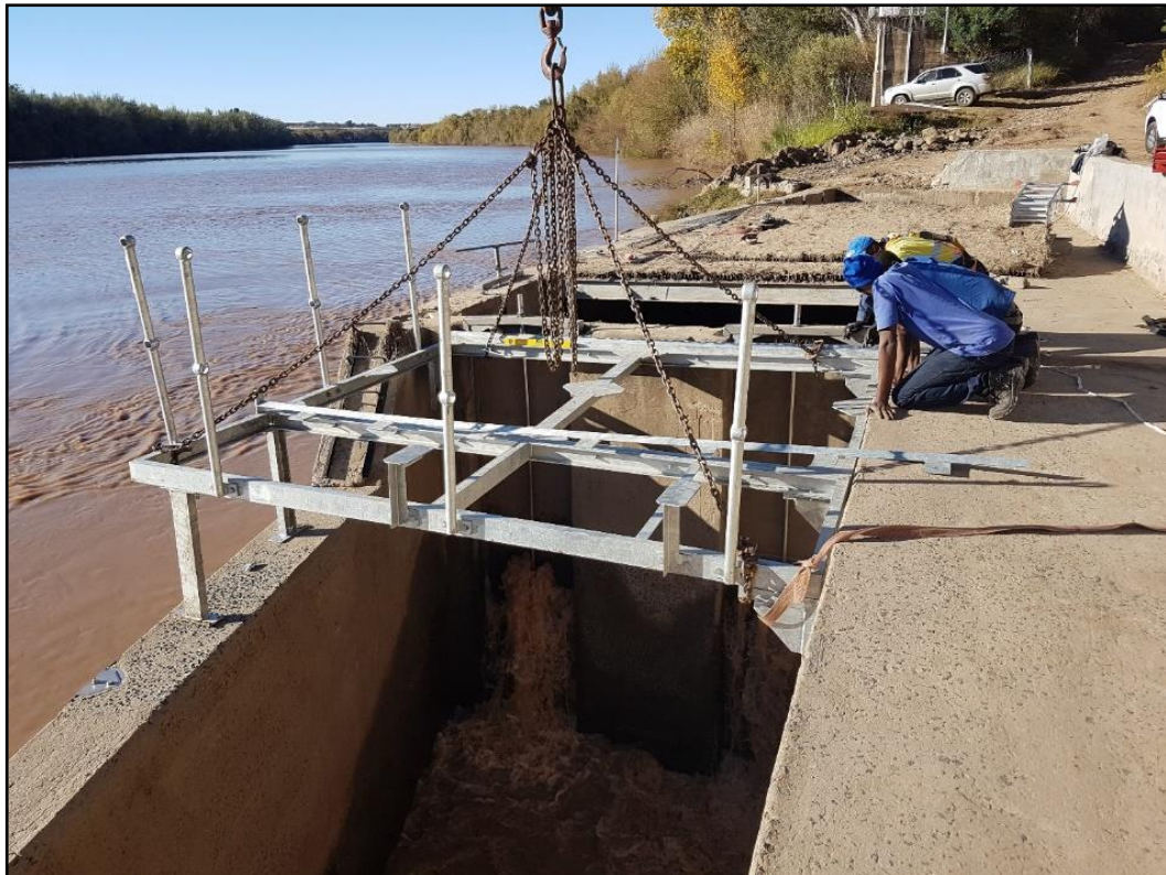
Figure D-3: New walkway frame in place
