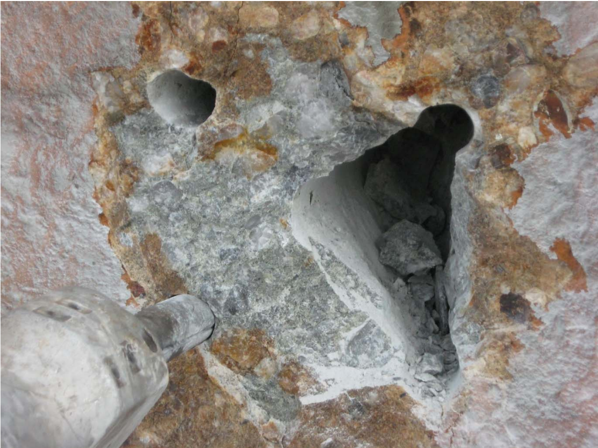
Figure 26:. Opening created with debris manually cleared (Author, 2013)
