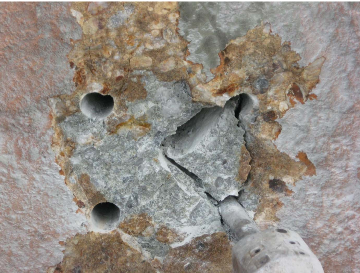
Figure 25: Fracturing during 5-hole trial (Author, 2013)
