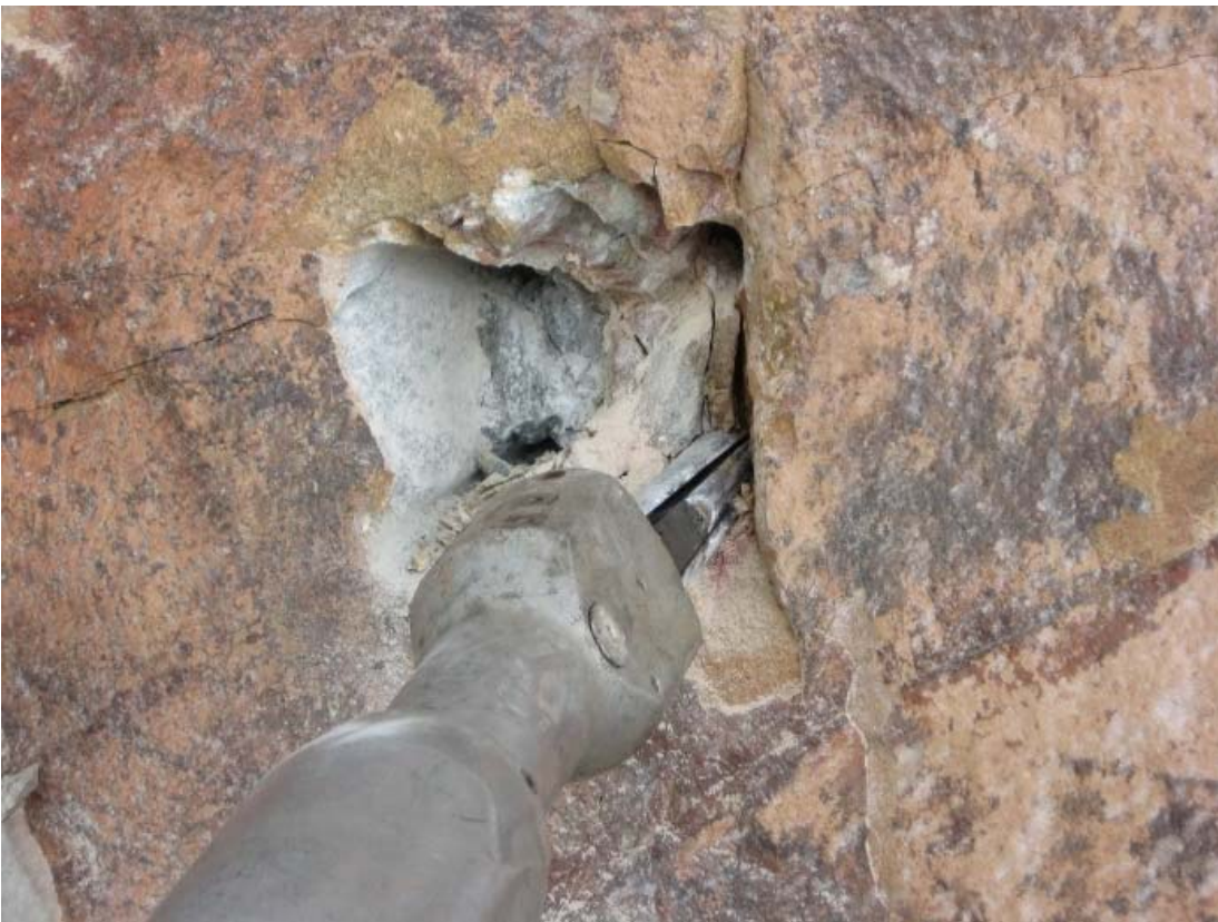
Figure 24: Progress made with the DARDA® hydraulic splitter (Author, 2013)
