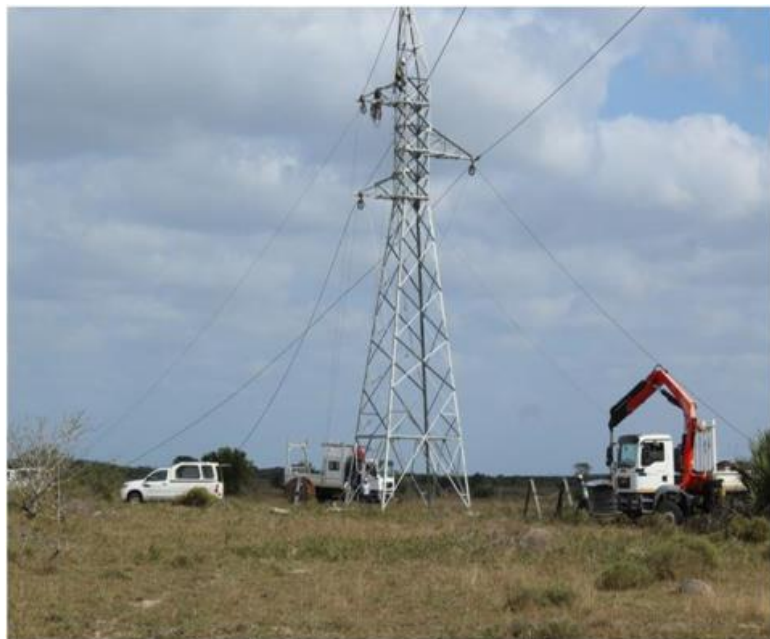
Figure 4.15 Stay supported structure
