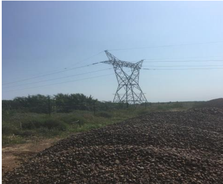
Figure 4.14 Waist-type self supporting tower source:
