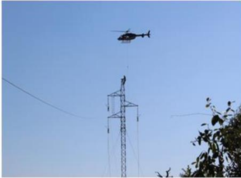
Figure 4.13 Helicopter stringing.
