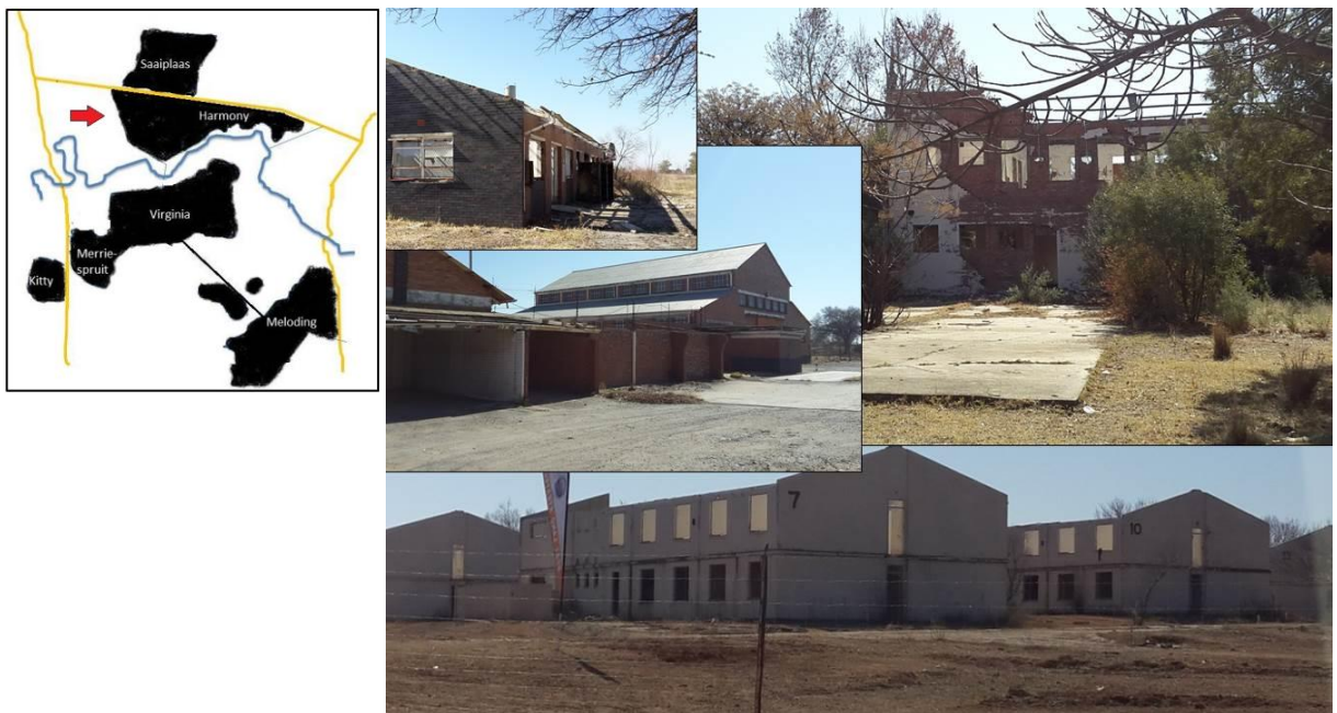
Figure 34: Derelict mine buildings, including offices, a hospital and hostels
