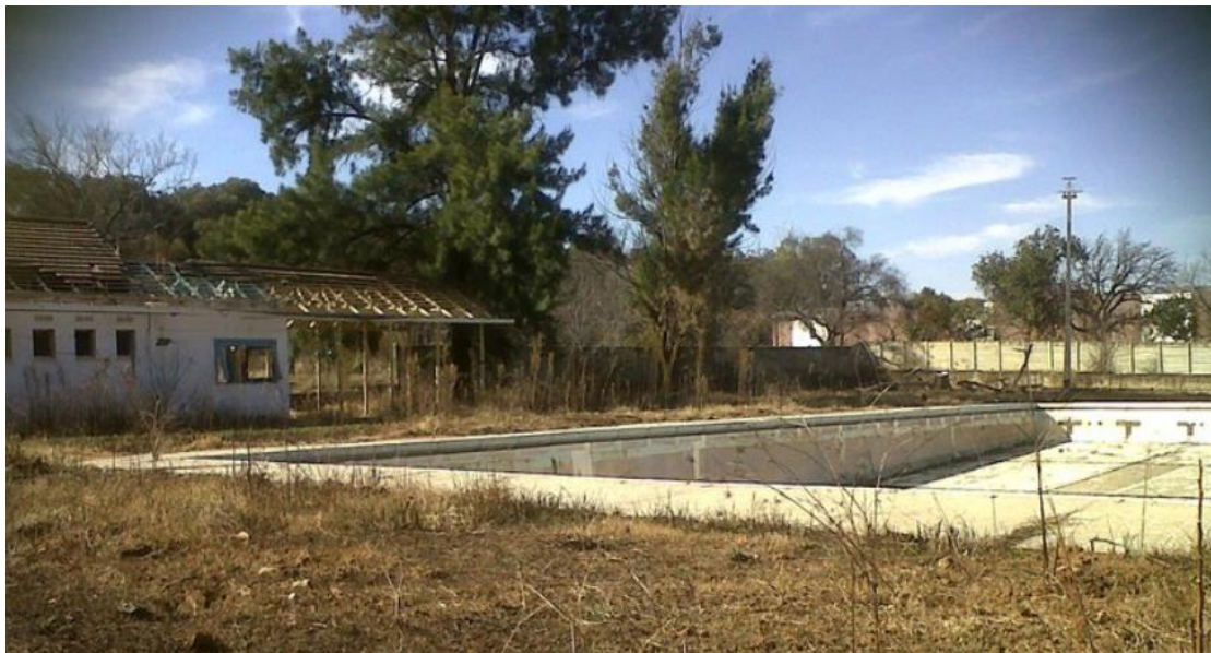
Figure 55: The Harmony Club swimming pool in 2011. Source: Fitzgerald, 2011
