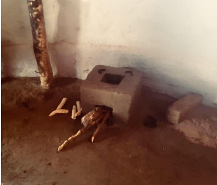
Figure 4-8: (b) Efficient stove during construction
