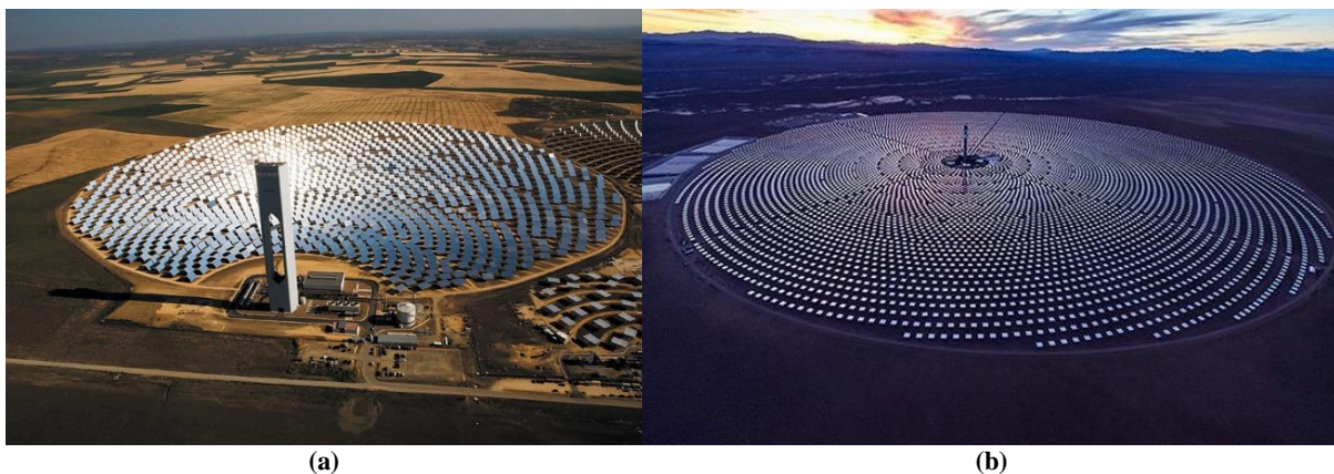
Figure 2.10: (a): The PS-20 north-facing heliostat polar field in Seville, Spain, is on the left (Wordpress.com, 2013); and (b): the Crescent Dunes surround field constructed near Tonopah, USA, on the right (Proud Green Building, 2017).
