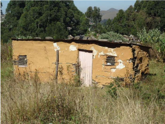
Figure 3.3: Building using stick and mud for wall construction at Msunduza
