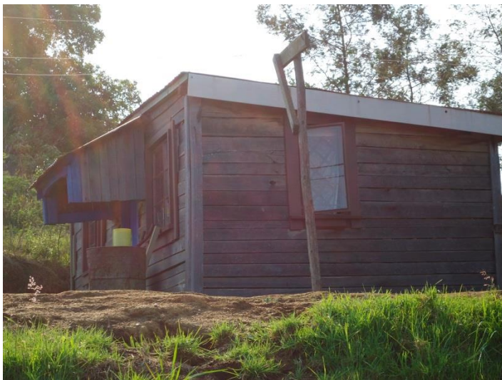
Figure 3.2: Building using wood panels as walls at Mahwalala
