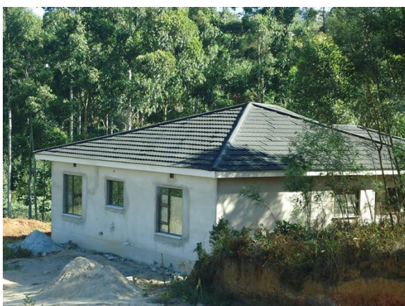
Figure 5.3: Concrete walled formal building with Harvey tiles for roofing at Mahwalala
