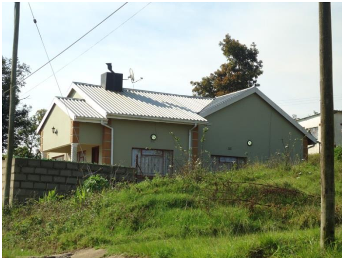
Figure 3.7: Formal building using concrete blocks for wall construction at Mahwalala
