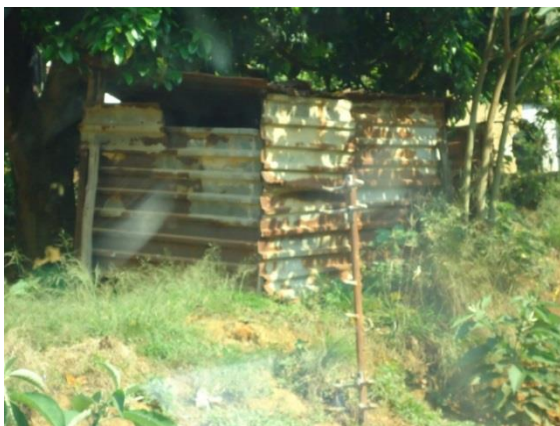
Figure 5.5: Pit latrine at Nkwadini
