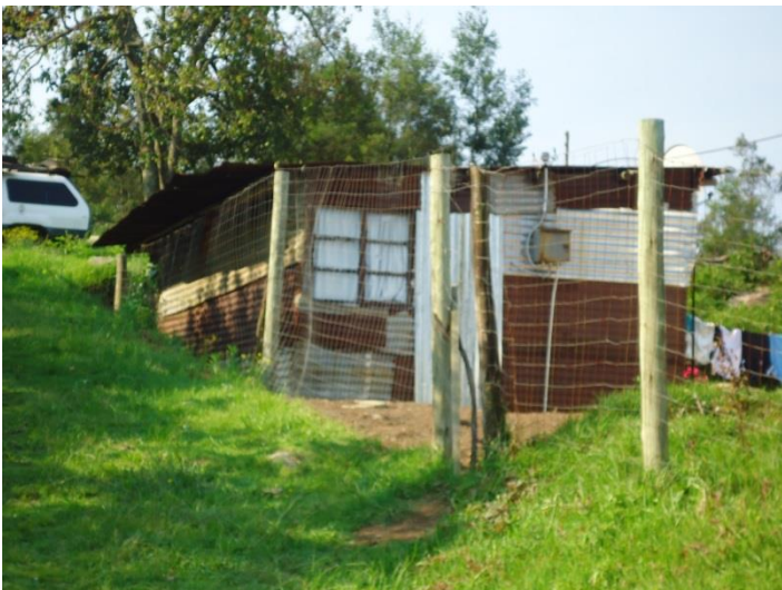
Figure 3.4: Building using corrugated iron for wall construction at Nkwalini
