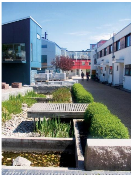
Figure 3.9: Drainage channel receiving water from the spouts and directing them to gardens. Photo by Ludwig, S.
