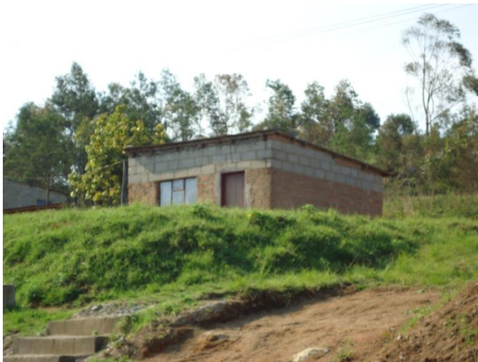
Figure 3.6: Building using combination of concrete blocks and compressed earth blocks for wall construction at Mahwalala
