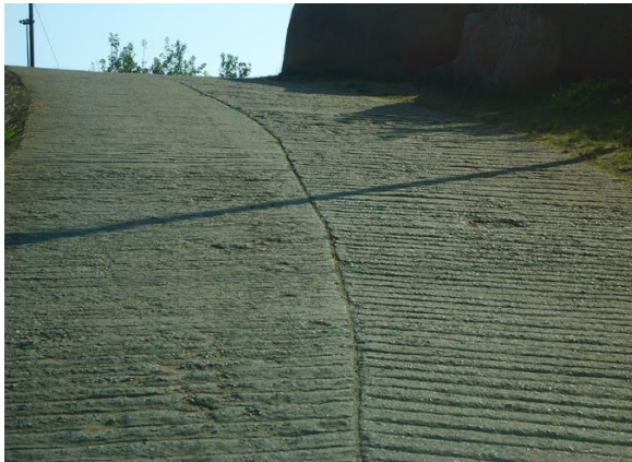
Figure 5.8: Concrete finished road
