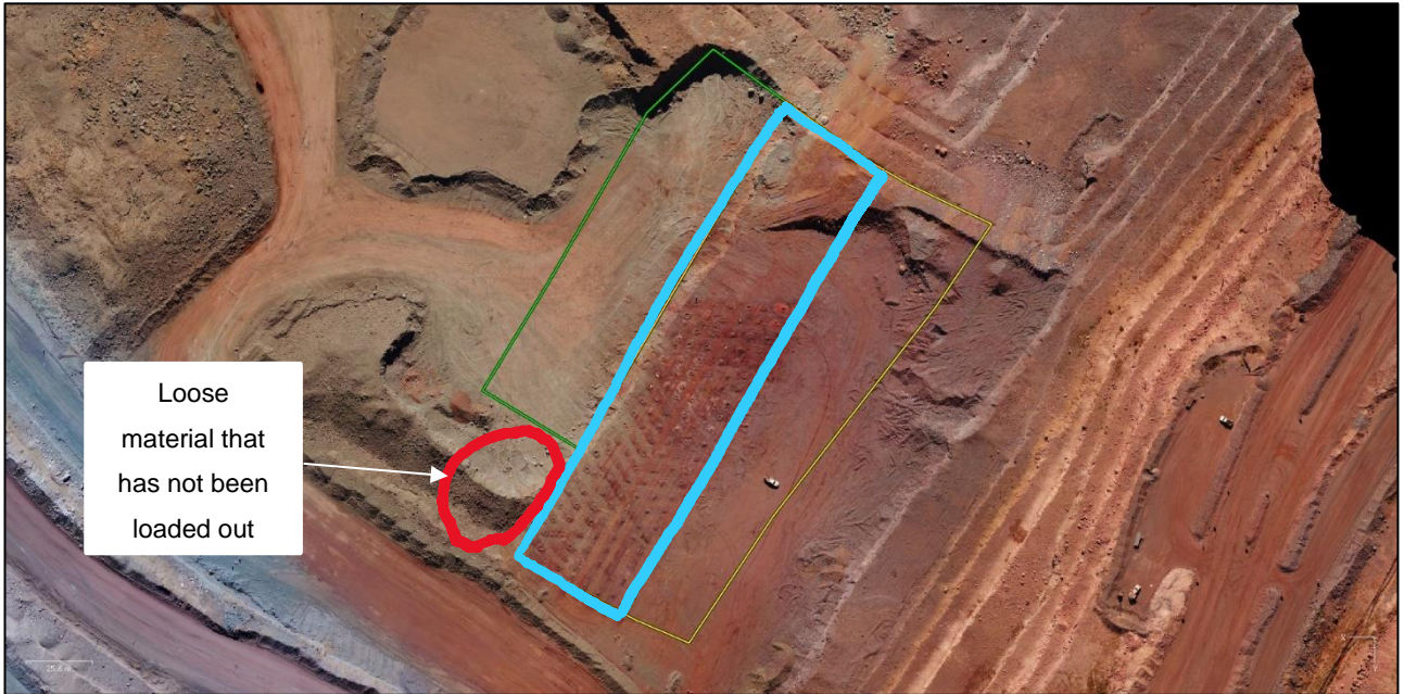
Figure 38: A view of the block on the day of blasting on 31 May 2018.
