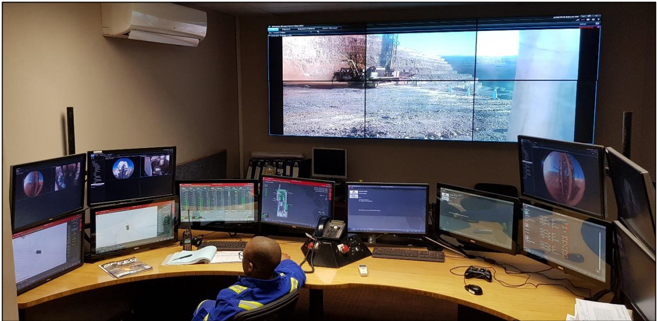
Figure 6: A view of the mines autonomous drilling control room.
