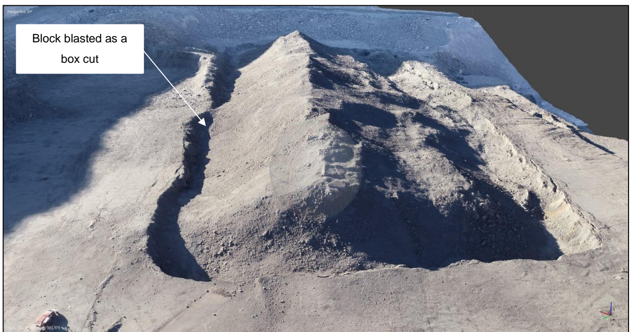
Figure 53: Block LFP1114O111 after the blast.
