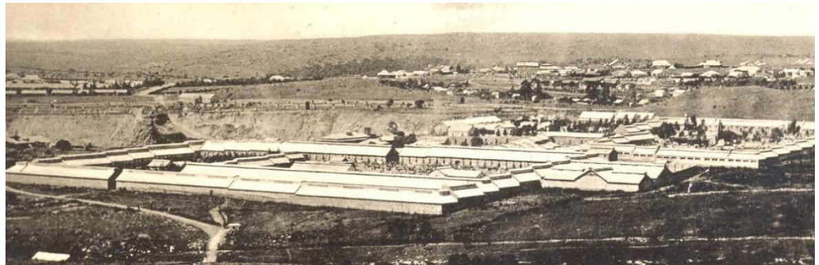
Figure 2.4 - Workers compounds - (Lincoln: 2011)
