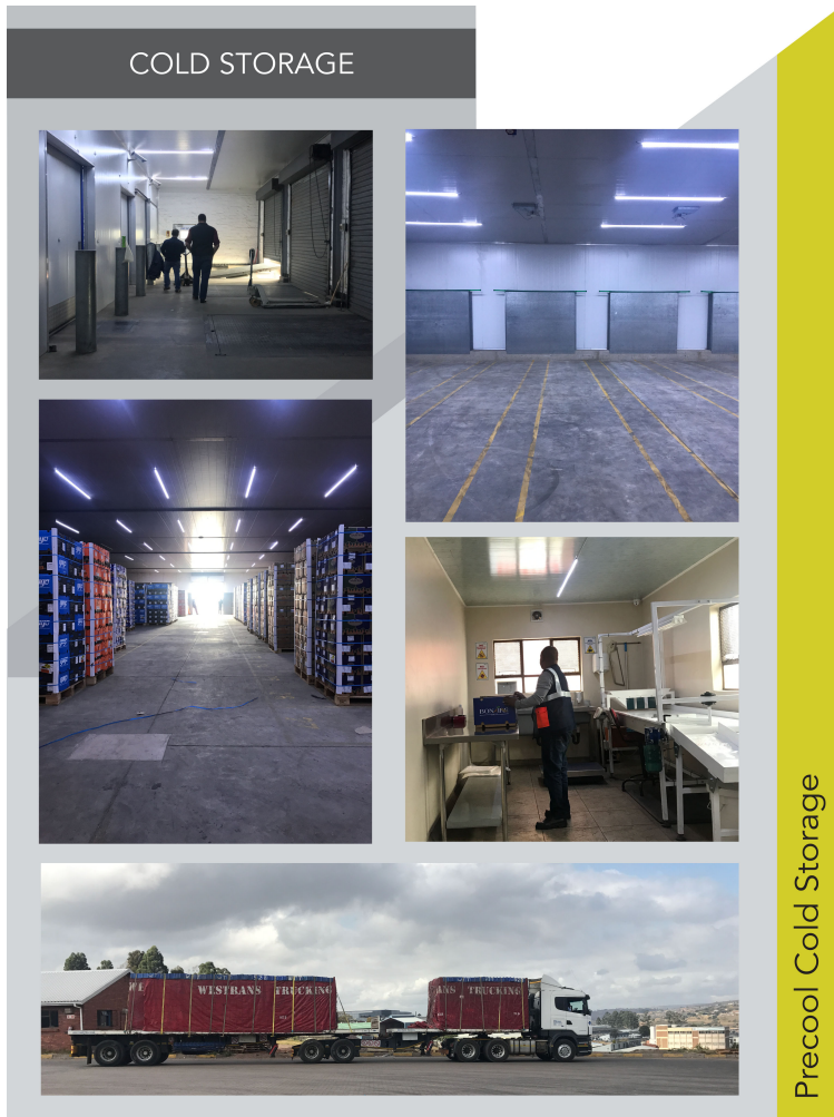
Figure 20 Precool Cold Storage facility
