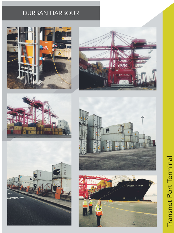
Figure 9 Transnet Durban Port Terminal
