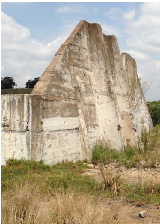
Fig. 2.12 Shaft No. 1 concrete walls (Author: 2018)
