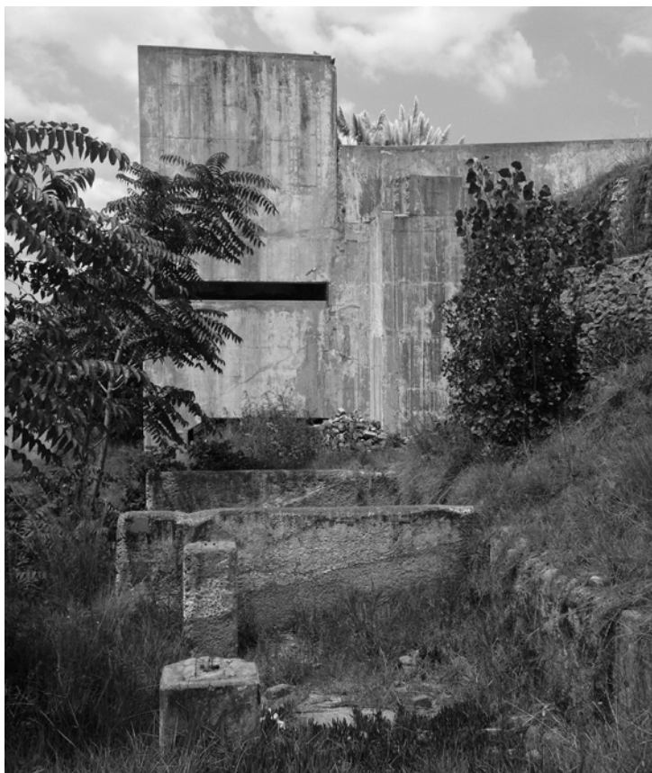
Fig. 01. Above; Village Main Shaft No 1 Remains (Author, 2018)
