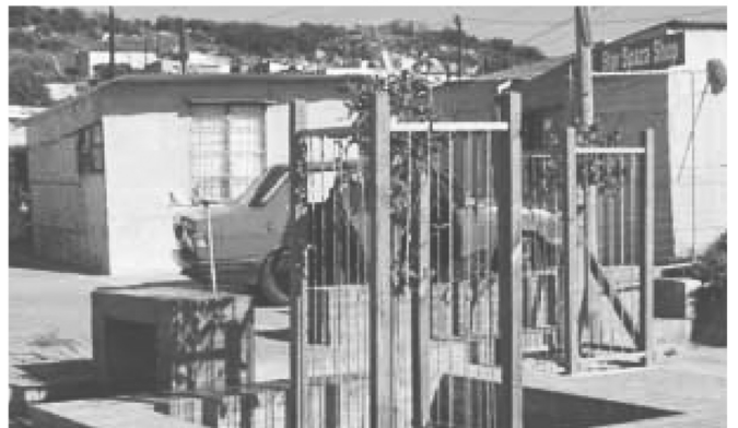
Figure 1.36: Completed Emthonjeni project. (VPUU 2016)
