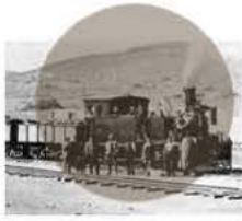
Delagoa Bay Railway Line built from maputo to Pretoria. First stop at Eerste Fabriek Station
