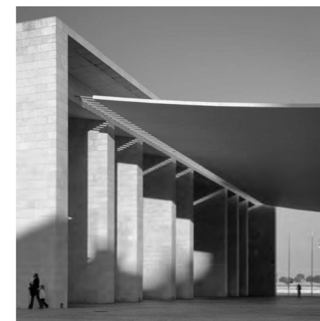
Fig. 5.3: (Left) Dramatic change in scale between two thresholds are marked with the two different concrete constructions of the canopy and portico. The two are connected with light steel members to express the idea of separation (Archdaily: 2015).
