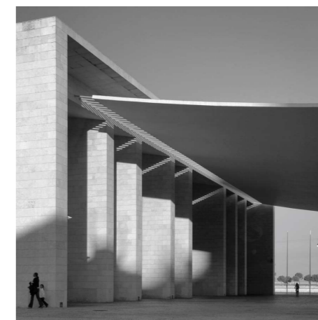
Fig. 5.3: (Left) Dramatic change in scale between two thresholds are marked with the two different concrete constructions of the canopy and portico. The two are connected with light steel members to express the idea of separation (Archdaily: 2015).
