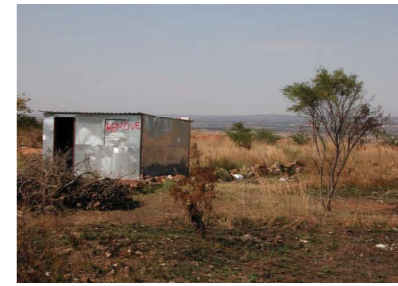
Figure 3.8 Illegal shack on the eastern ridge. There is an attempt to halt and manage the spread of illegal housing on the mountain; note the "remove" sign on the shack (Maree, 2012:30).
