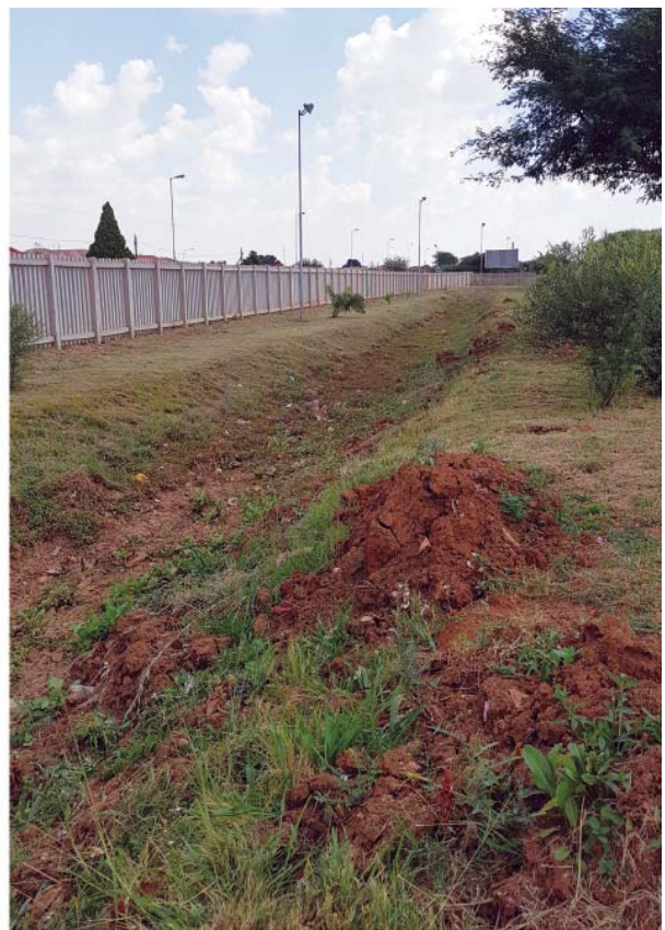
Figure 6.117 Below: Current storm water swale (grassed lined channel on site (Author 2018).
