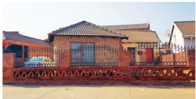
Figure 5.71 An example of a patterned boundary wall, using brick in Mamelodi (Author 2018)
