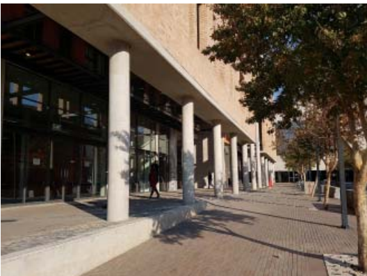
Figure 3.60 Sol Plaatje University, edge of Building CX003 to the public square. Deep threshold spaces allow for shading of the building interior, which faces west (Author 2018).
