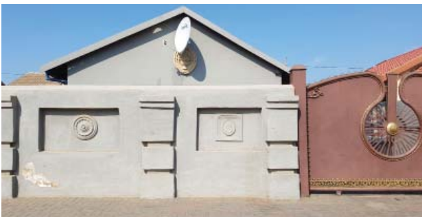
Figure 5.70 An example of a patterned boundary wall, using plaster, paint and steel work from artisans in Mamelodi (Author 2018)
