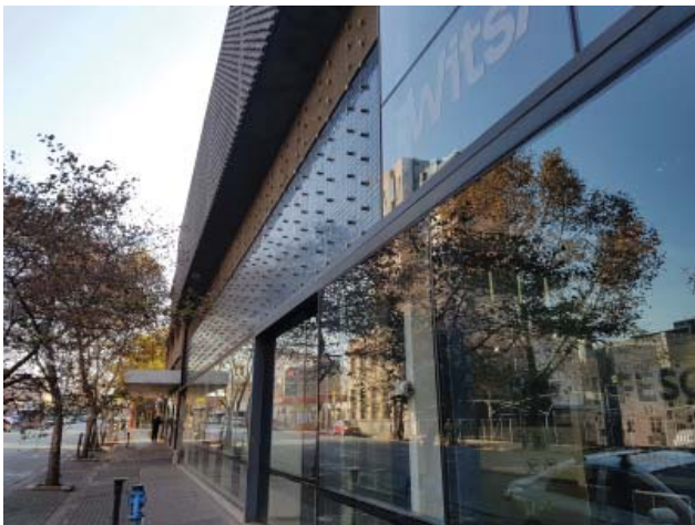
Figure 3.66 Clear glass between the street edge and the interior coffee shop allows for visual interaction.
