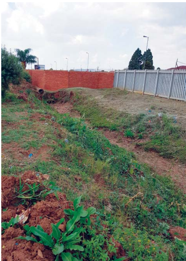
Figure 6.117 Below: Current storm water swale (grassed lined channel on site (Author 2018).
