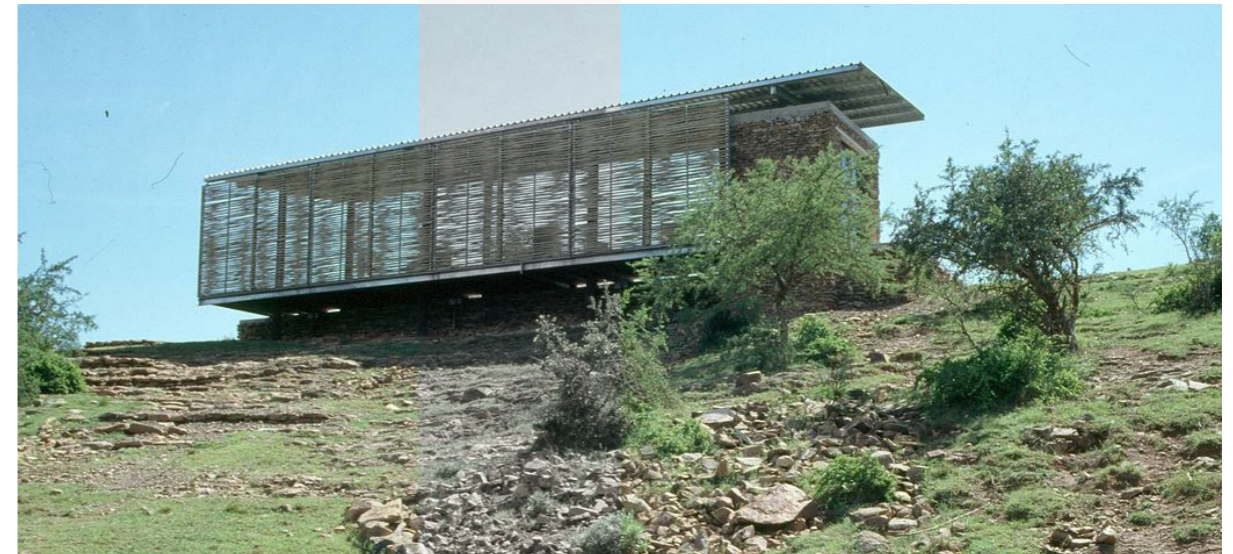
Figure 3.16 The Nelson Mandela Museum structure (Cohen and Garson, 2018)
