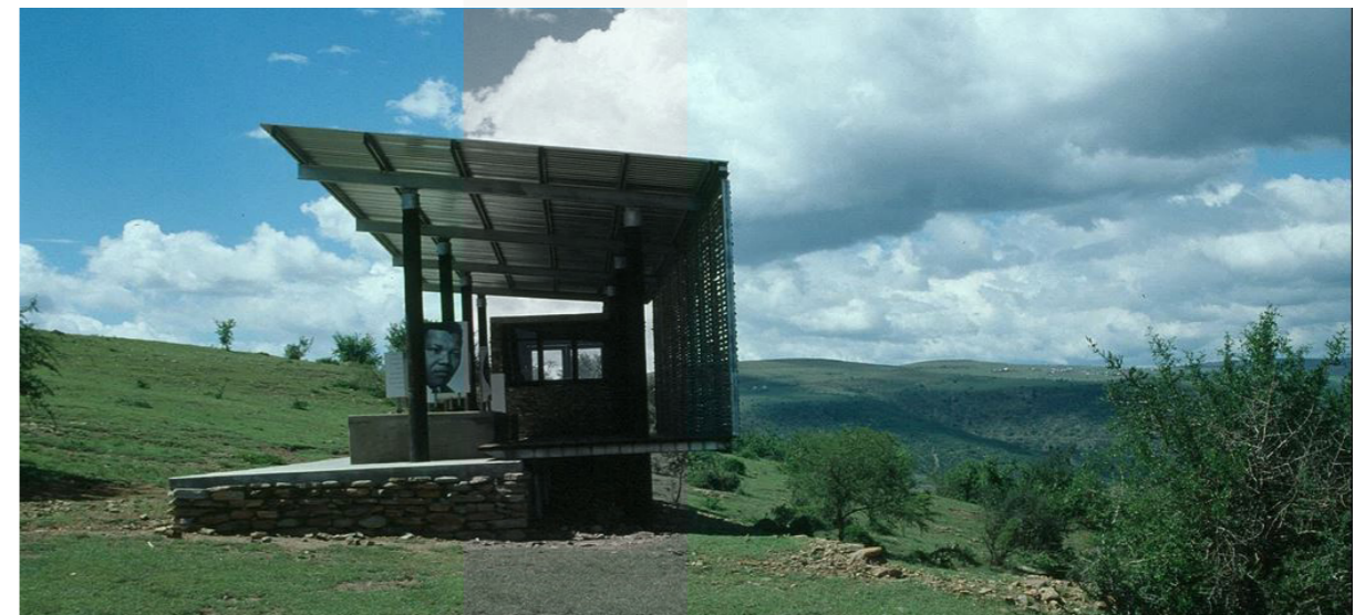
Figure 3.17 The Nelson Mandela Museum structure (Cohen and Garson, 2018)
